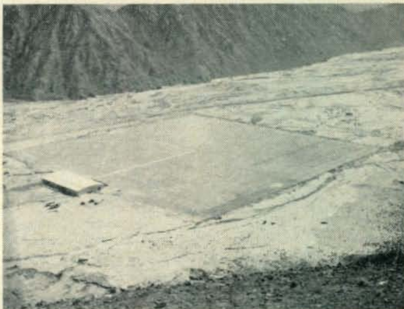
Here's the giant antenna we were talking about last month. Located on the equator near Lima, Peru, at Jicamarca Observatory, what you are looking at above is 9,216 crossed-dipole elements. It is utilized in a method known as scatter radar for studying the ionosphere and exosphere.
