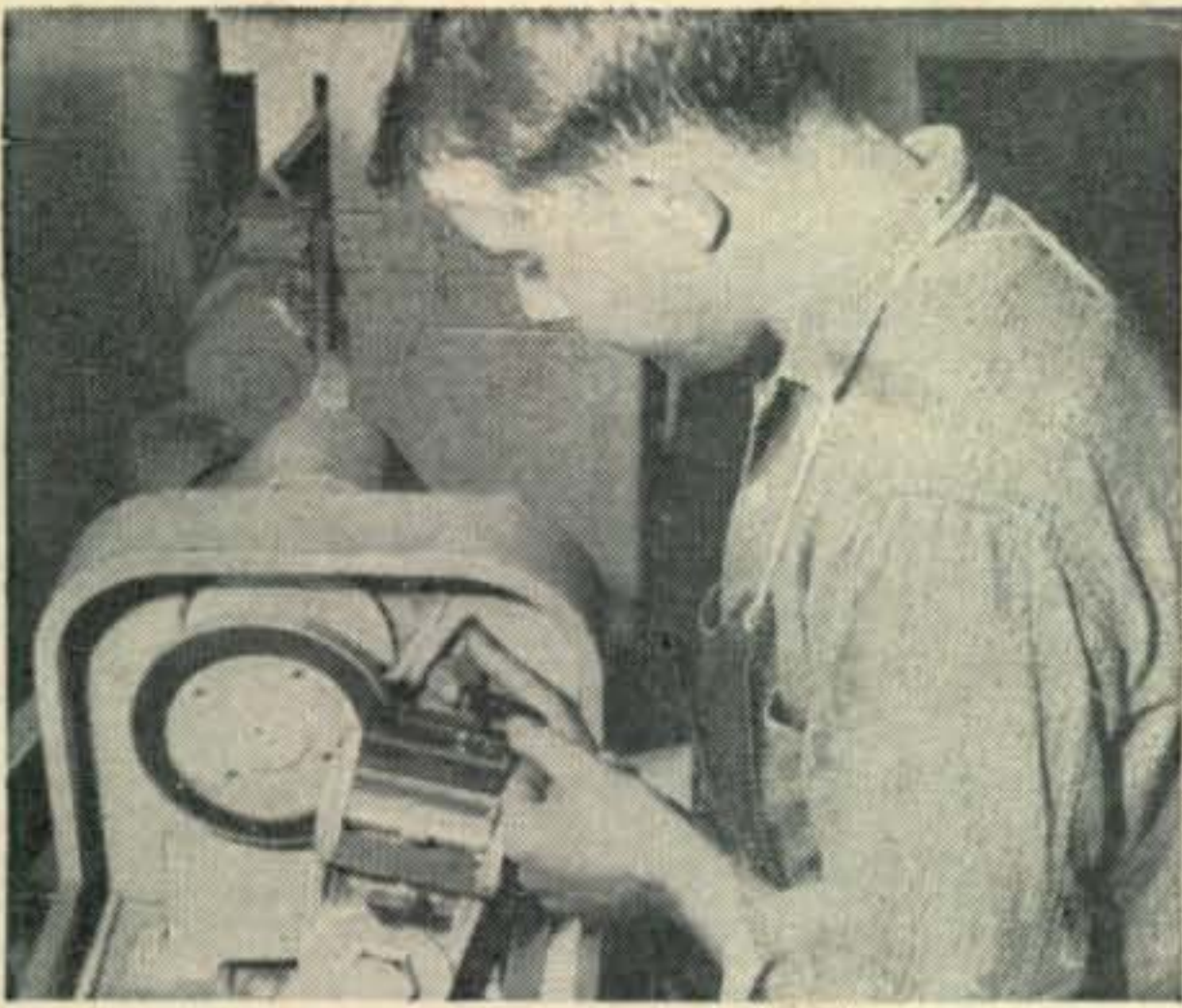
Edging, Rounding and Pre-dimensioning Blanks.
