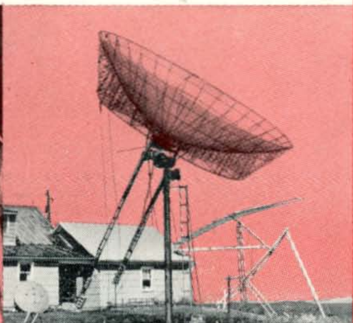
Moonbounce antenna — the 27-foot diameter parabolic dish built by Mr. Vic Michael, W3SDZ, of Williamsport, Pa.; a measure of the initiative and dedication of moonbouncers.
