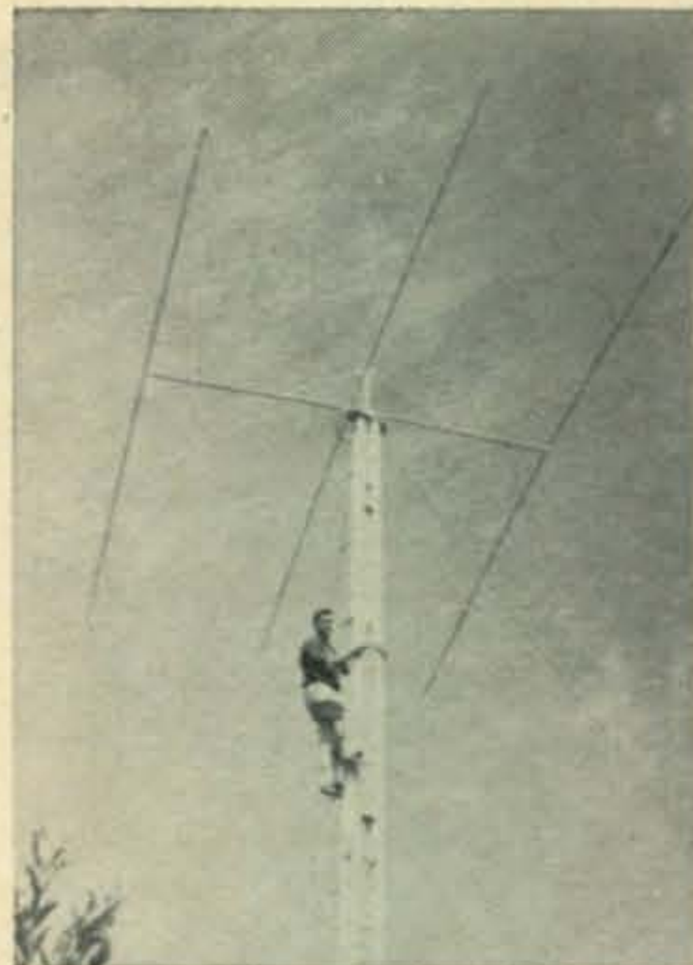
Tom, nearing the top of the tower which held a Hornet beam whose 20 meter capabilities were impaired by a broken tip on one of the elements.
