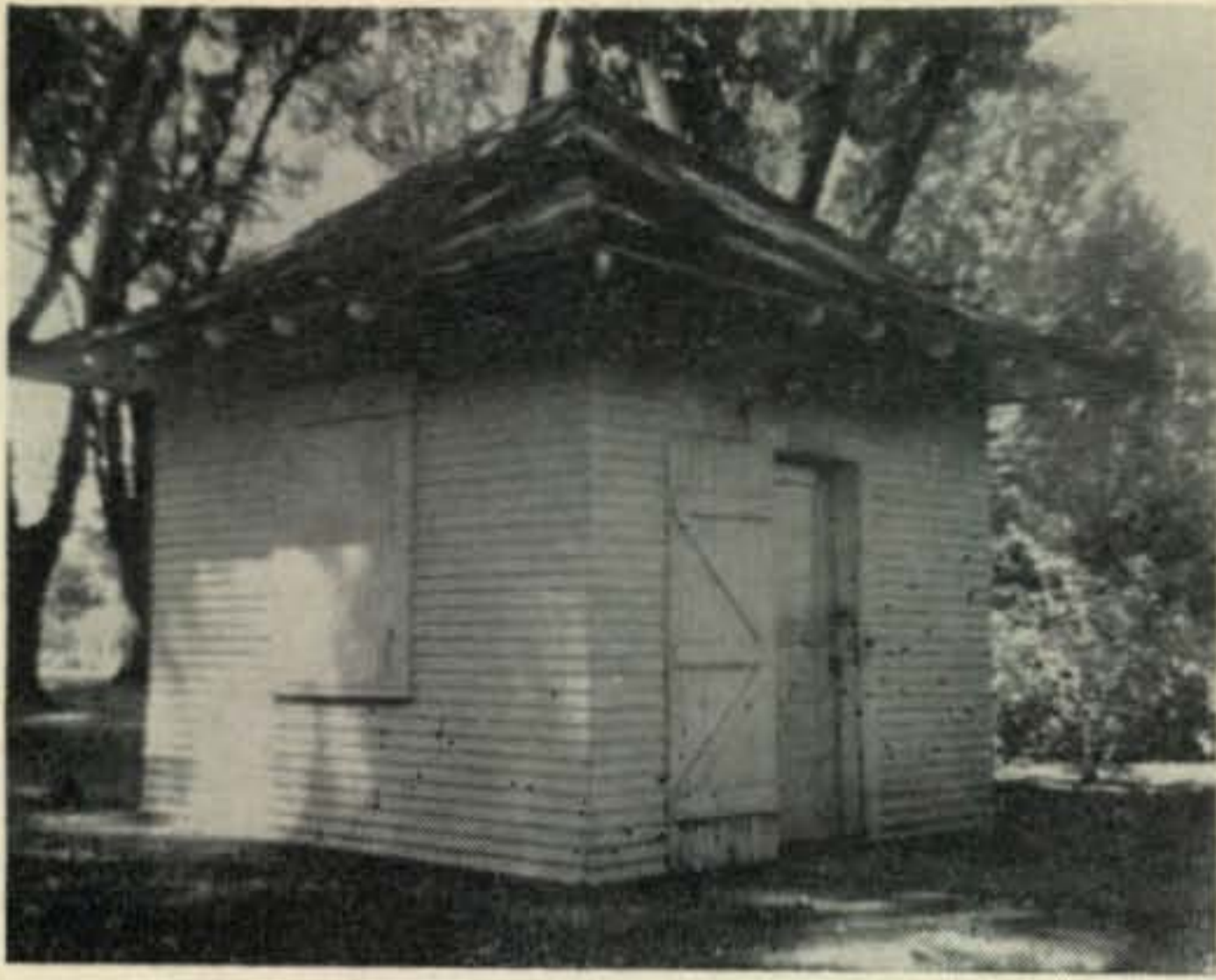
Pioneer hams were not the only ones housing equipment in detached buildings. Shown above is the radio shack used by the United Wireless Telegraph Company in Walla Walla, Wash., in 1908-1909. It now serves as a storage shed for garden tools in the Walla Walla City Park.
