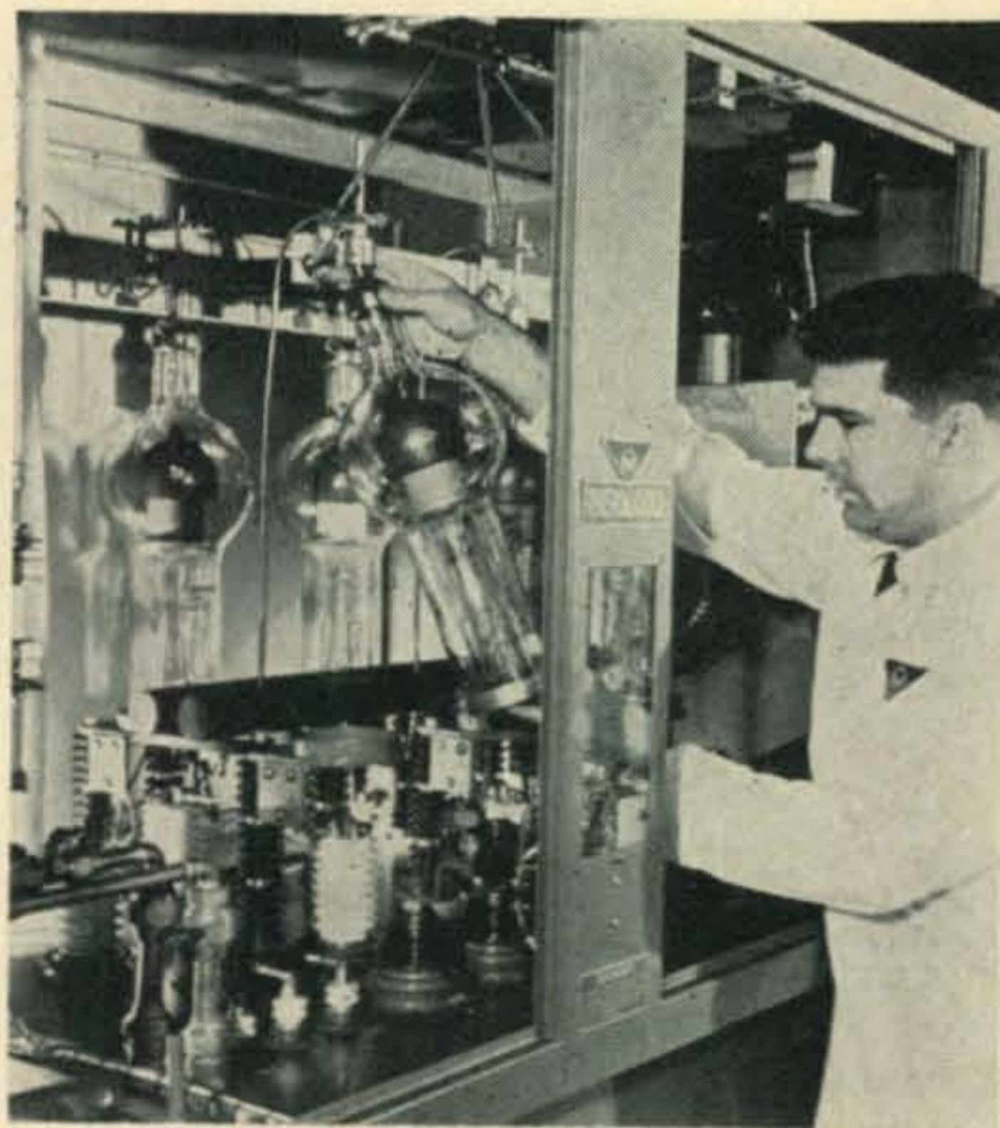
This could be Jess, K2EEM, putting the finishing touches on the big rig for 20, but it's not. Jess is shown at his job with AMF completing a 280 kw welder. For those of you who are spec conscious, the welder will permit continuous welding of half inch thick steel pipe up to two feet in diameter at speeds of up to 42 ft. per minute.
