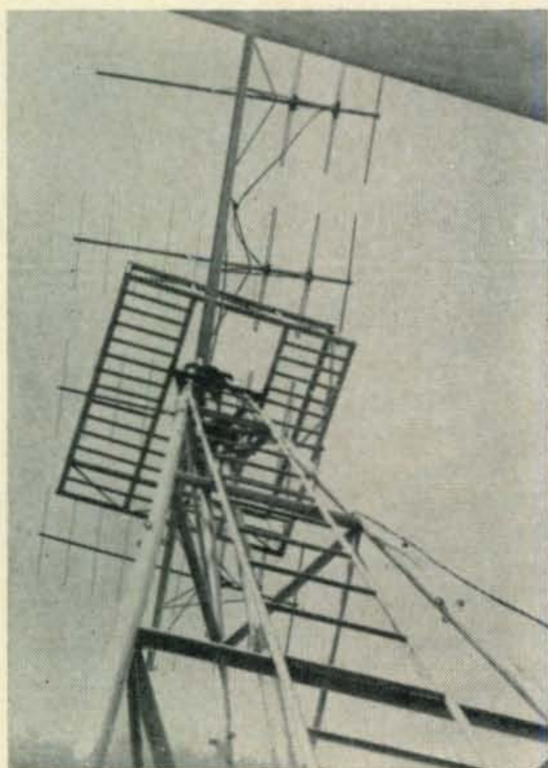
The array of Yagi antennas used by CR6CH to receive ESSA-2 APT transmissions on 137.500 mc.
