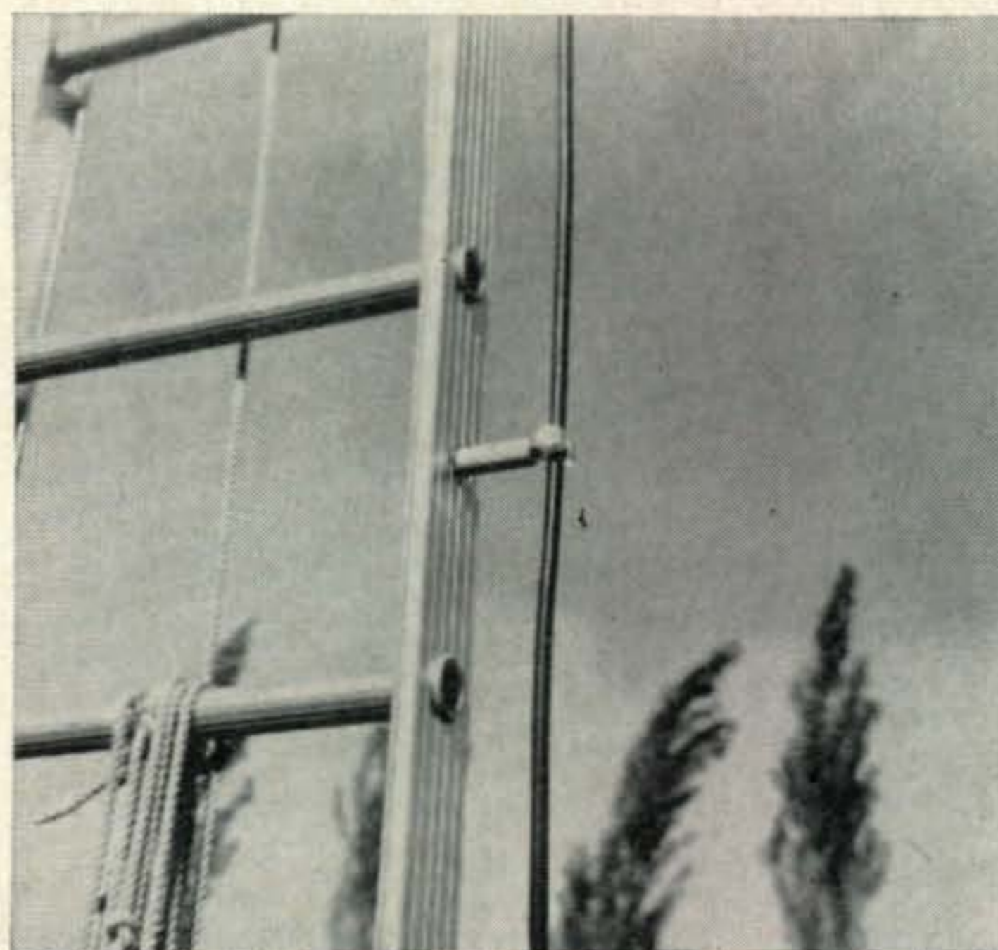
Close up of the coax line secured by the spring steel clips.
