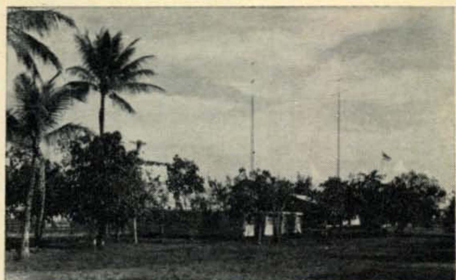
W0GTA/8F4—Bob Snyder's beautiful location at Pekanbaru, Sumatra. The 10/15 beams on left tower, 75 ft. up and the 20/40 job at right on a 90 ft. tower. All were 2 el. yagis. Bob had a 144 ft. vertical for 80.
