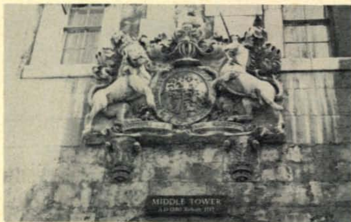
"There's a lot to be said for an old house. . . ." (Tower of London)
