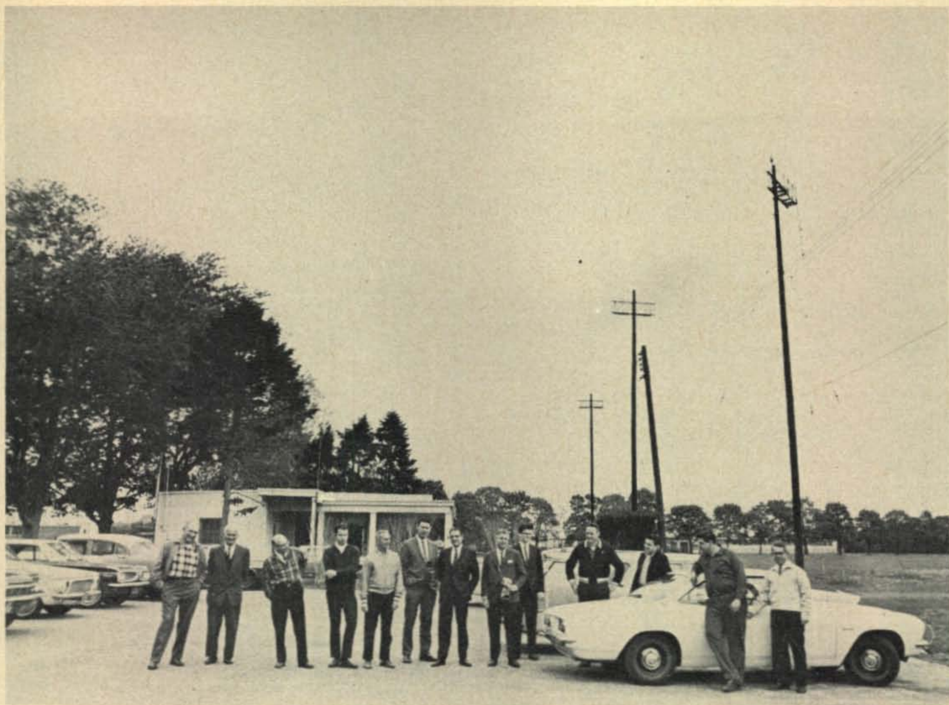
General view of NASTAR Headquarters shows some members with the shack and three of the 80 foot antenna poles behind.
