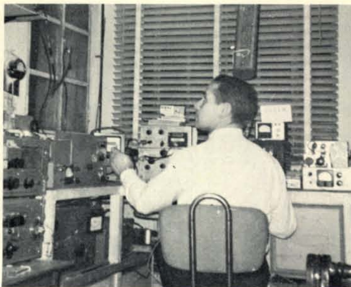
Lito, LU2EW shown tuning-up his home-brewed two meter station with which he plans to communicate through OSCAR satellites from his QTH near Buenos Aires.
