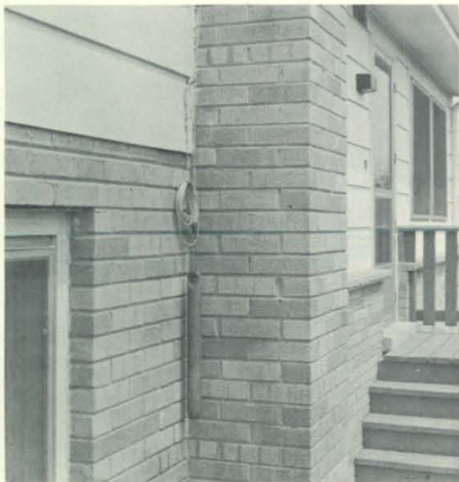
Fig. 4—The antenna is kept under constant tension through the use of a sash weight as shown above.
