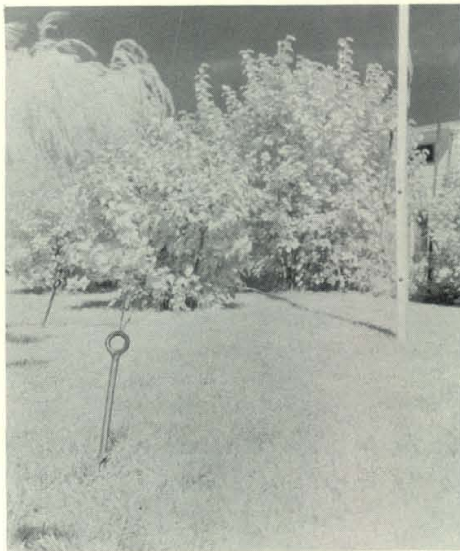
Fig. 3—A close up of one of the anchors used to hold the guys in place. A second anchor may be seen in the left background and the mast is on the right.
