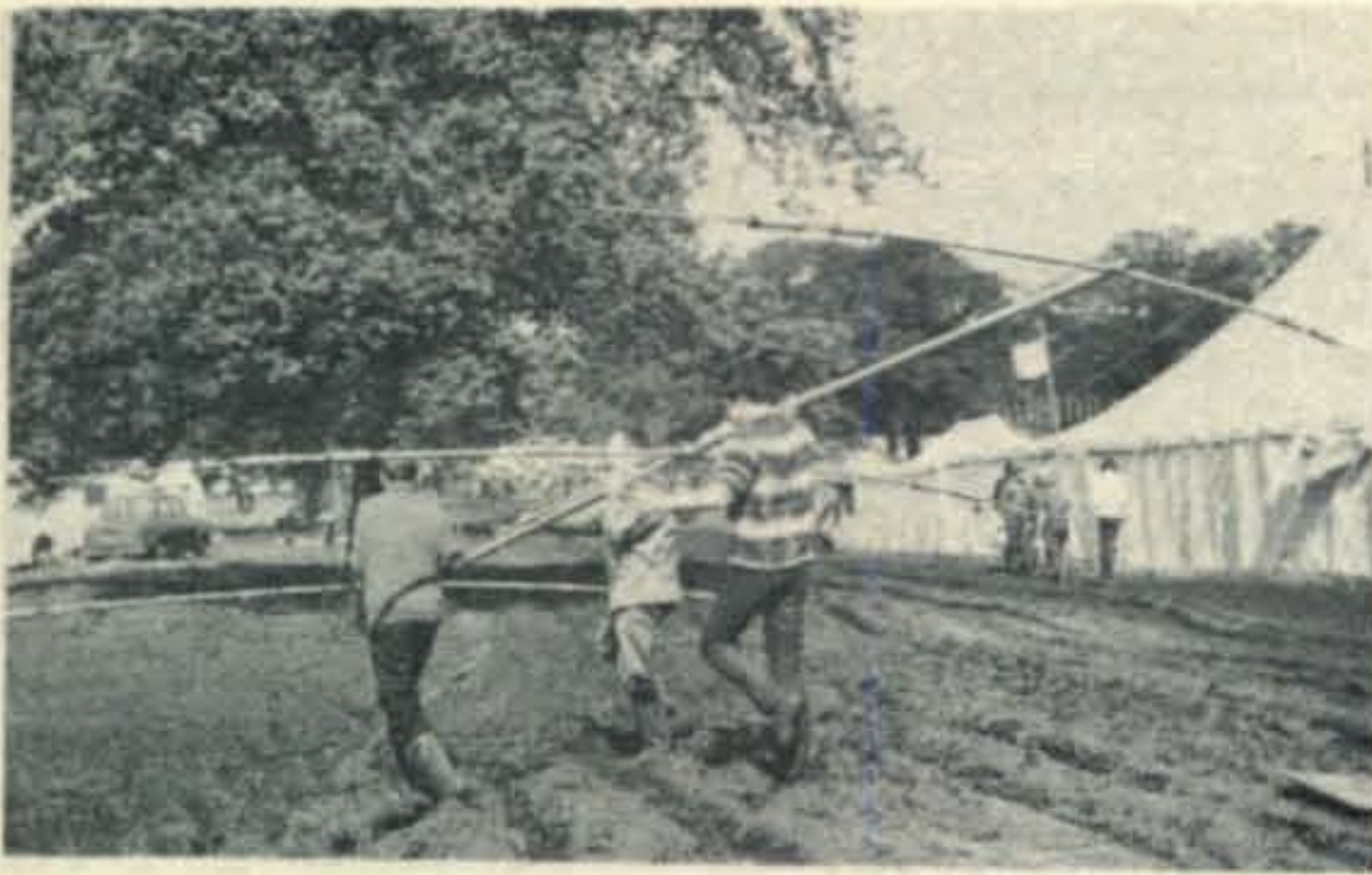
Up goes the beam out of the 15-inch-deep mud.
