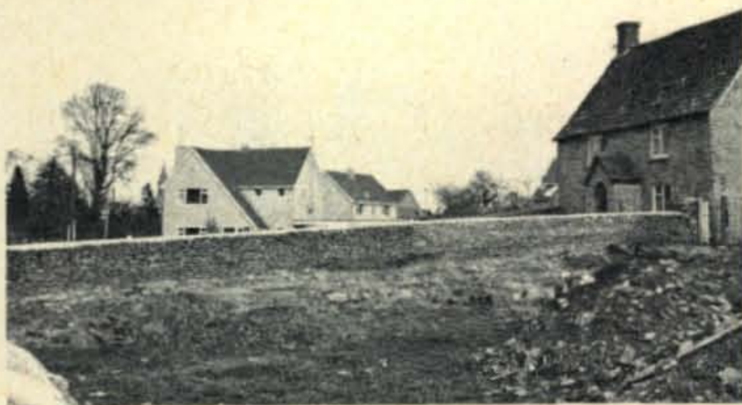
15th century cottage on right, modern home on left. Note dry-stone walls, local specialty which pioneers took with them and used the skill in some New England villages.
