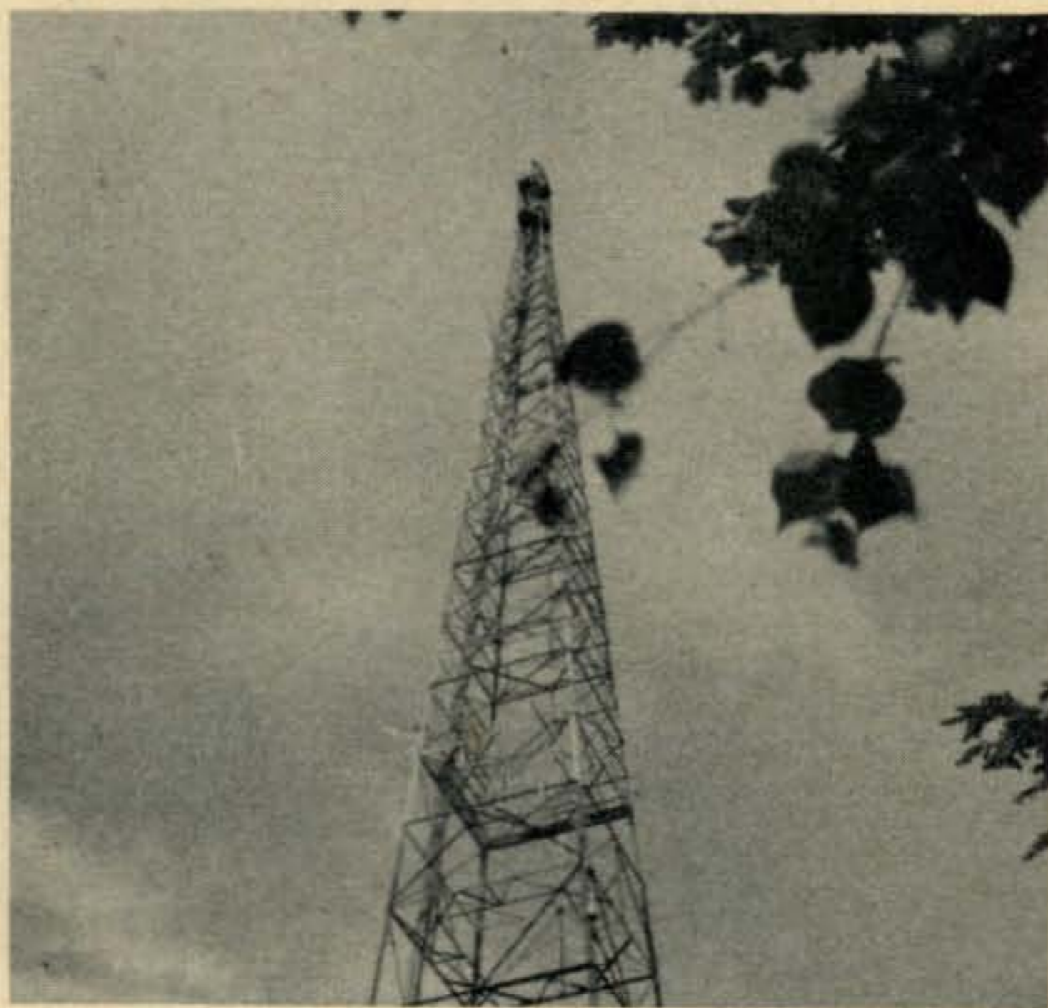
The 160 meter antenna support at W1DEO. The 325 ft. tower on a hilltop supports Herb's 265 ft. semi-vertical antenna.
