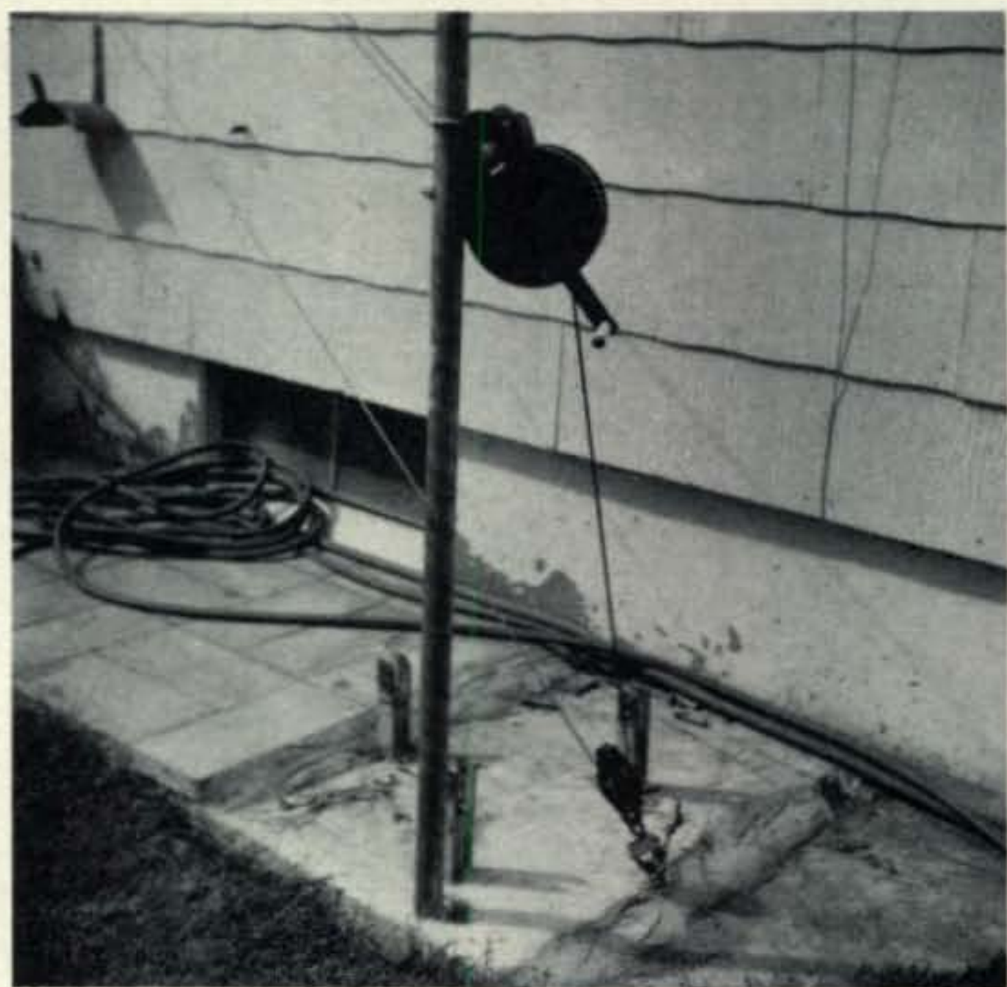
Fig. 3—A 1600 pound double locking boat hoist from Sears Roebuck does the job, along with 3/16" galvanized cable, a 750 lb. pulley, and a 1/2" eyebolt in 4 feet of concrete.
