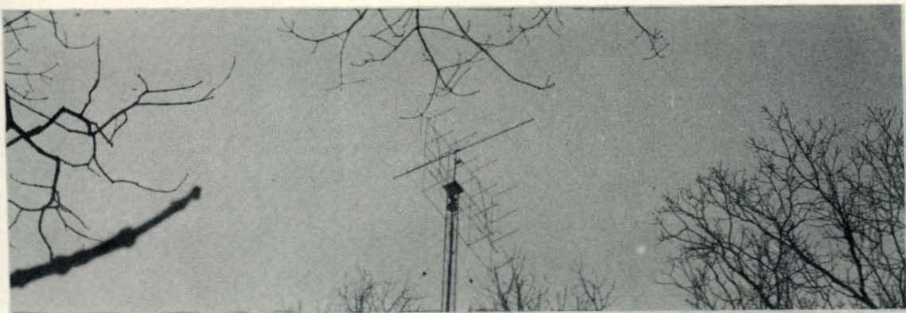
A 14 foot single 2 meter yagi atop sixteen 3\frac{1}{2}' 432 mc yagis at K2UYH. These antennas are topping a 100 foot tower.
