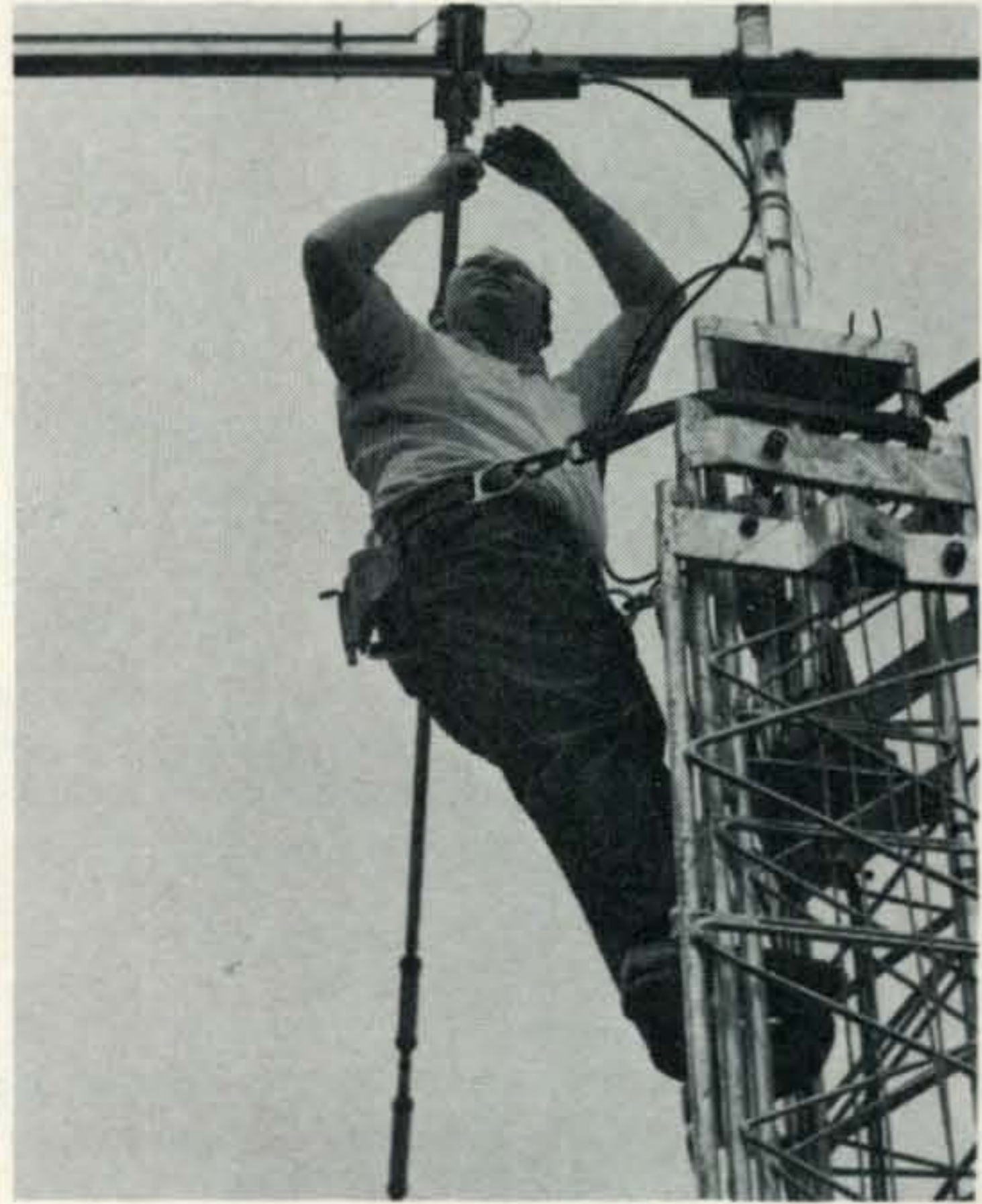
The 4-foot piece of pipe clamped to the end of the tower will support a 40 and 80 meter inverted vee antenna. Pully and lanyard for hoisting that antenna up and down are already affixed.
