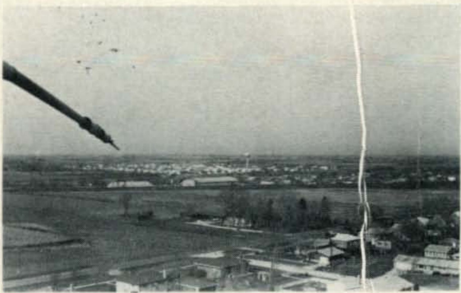
We see many photos looking up at beams and towers but here's one looking from the top down. It was taken from the "crow's nest" at the 120 ft. level of W9 EXE's tower.
