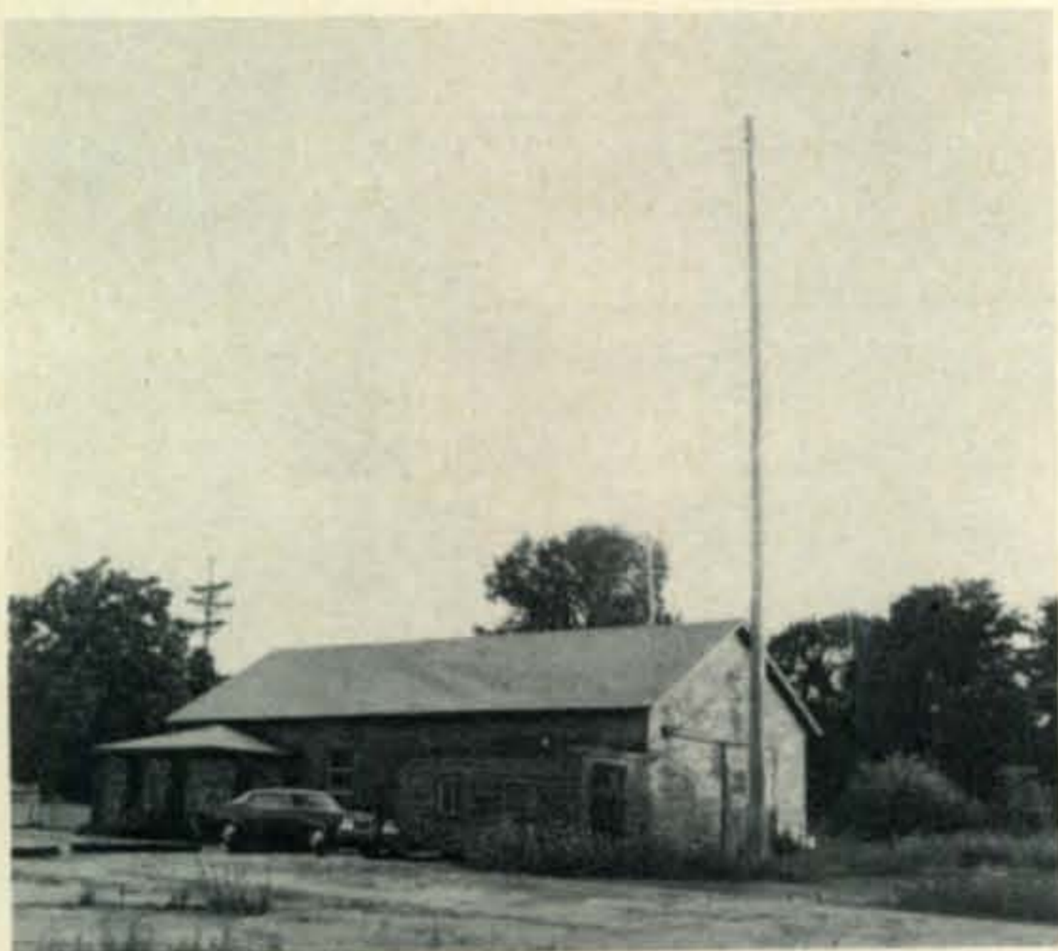
The antenna installation of the La Porte, Indiana, 146.22/146.82 mc repeater is a 90' telephone pole with pipe extension. The physical location is the old State Highway Barns, now part of Concord Corporation.
