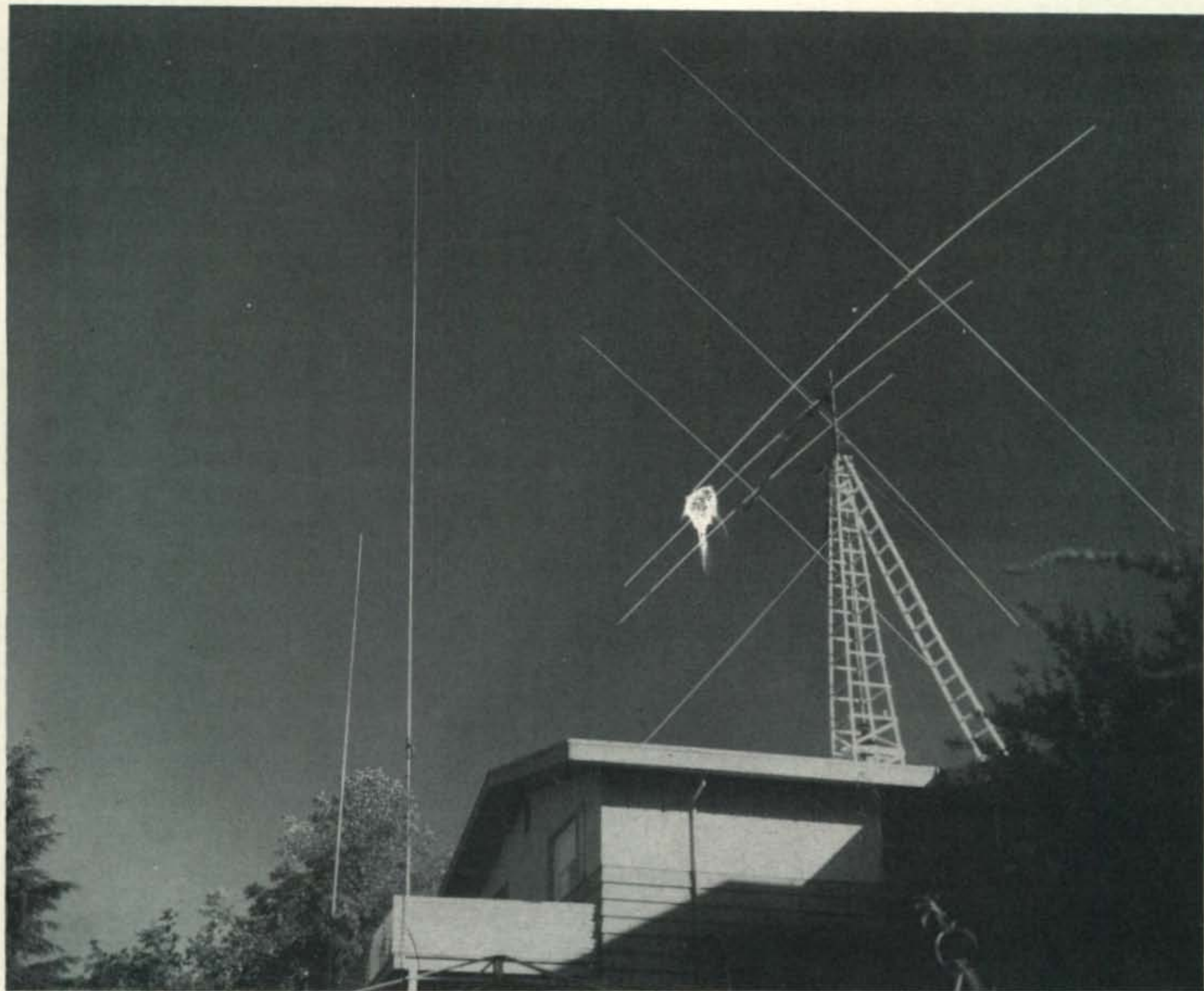
Half-wave antennas for 15 and 20 meters are mounted at opposite ends of a sun deck with minimum interference to each other or to the beam.
