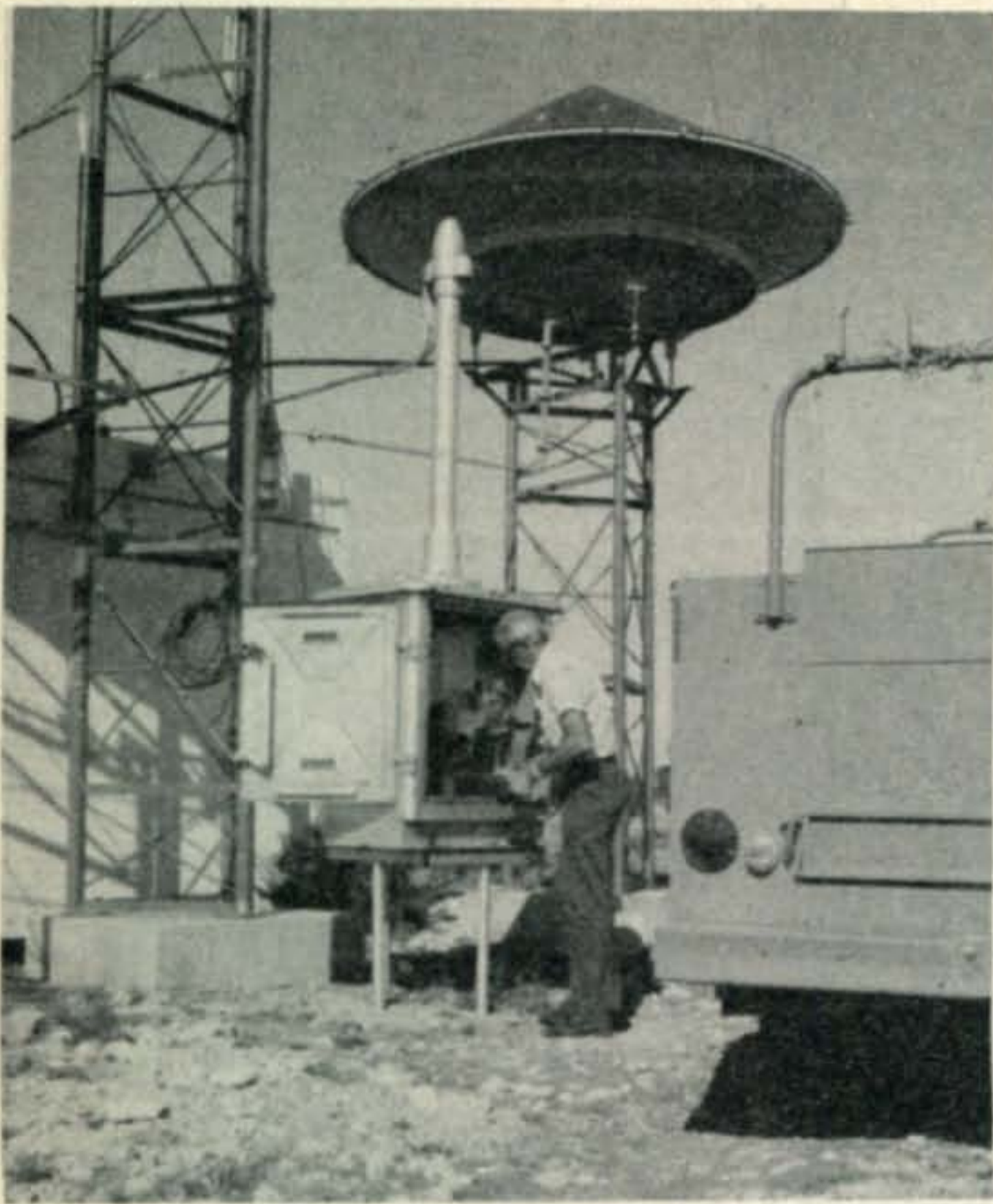
Alex, W5TOC, shown checking out W5AW, the Big Spring repeater. Repeater site is about 2 miles south of the city on a hill. The receive antenna is a "J" pole about 250' above ground. Transmit antenna is about 220' up. (Photo courtesy of WA5KHU)
