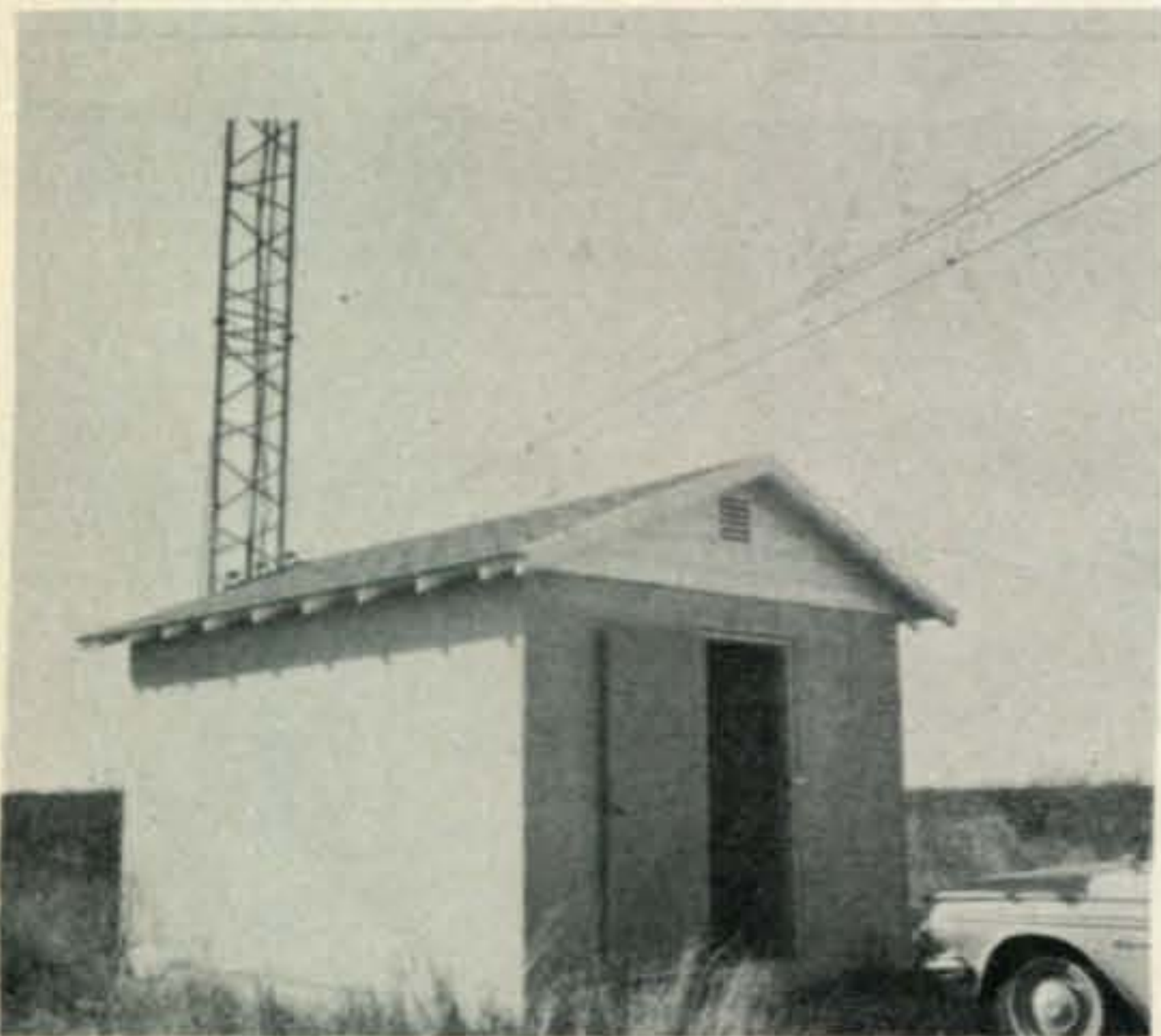
Site of Midland, Texas repeater is about 4 miles south of the city. The receiver antenna is a DB-220, 360' above ground and the transmit antenna is a 5/8 wave groundplane 300' above ground. (Photo courtesy WA5KHU)
