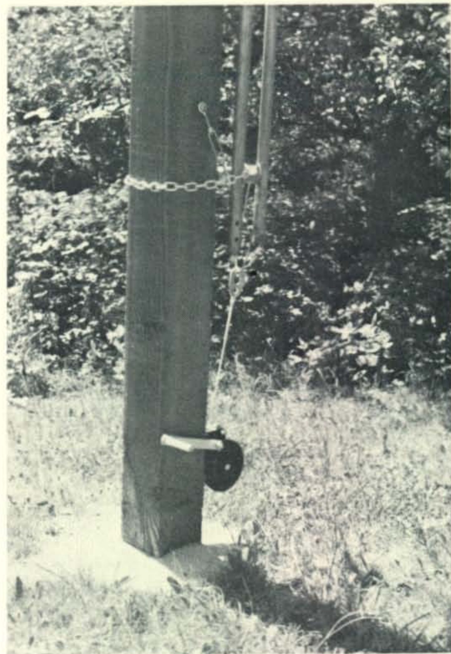
A double-ratchet boat winch bolted to the bottom of the timber allows easy raising and lowering of the tower. Note the chain used to secure the tower against curious children.
