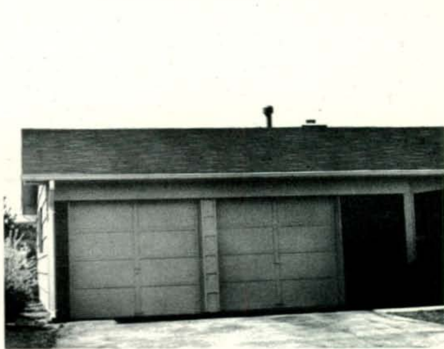
Fig. 5—The disappearing antenna of WA3HDU. By means of a clever hoisting mechanism, WA3HDU lowers his beam below rooftop when it is not in use.
