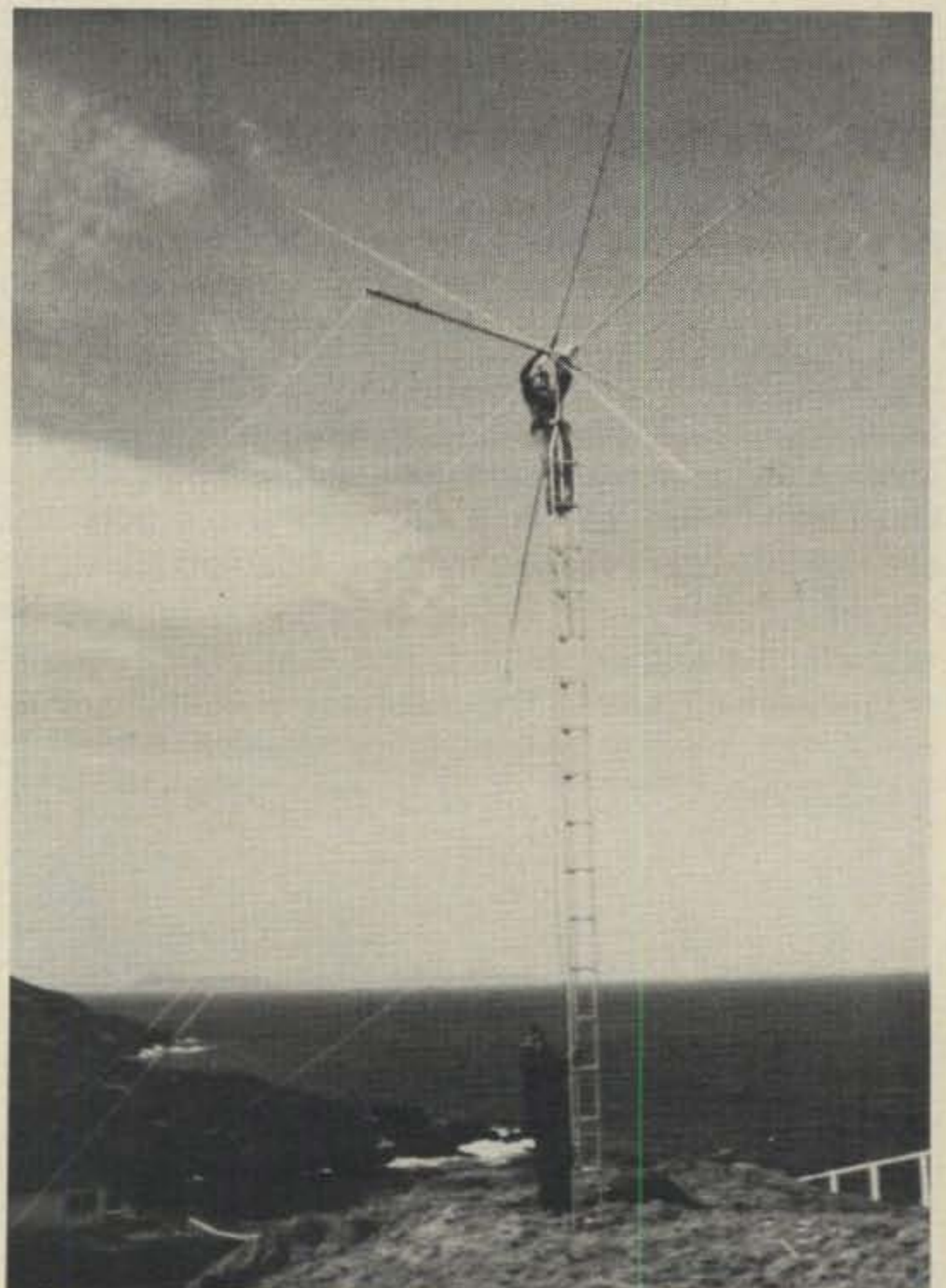
VE3BMV installing the "tail" on the Quad, while VE3DU is trying to shake him off. The rotator had to be replaced with piece of pipe and rope.
