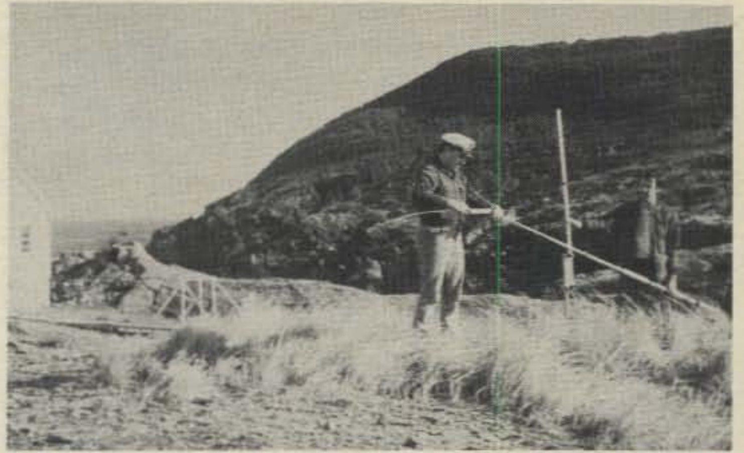
The 18AVT being assembled and installed by VE3BMV and VE3BBH.
