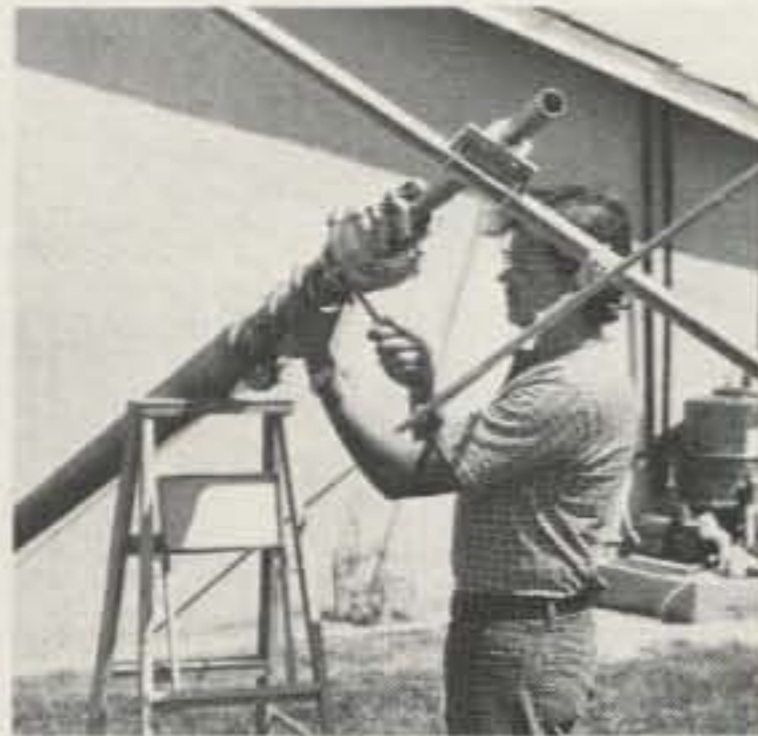
Hinged Base Plate allows tower to be lowered for access to antenna and rotor from the ground.
