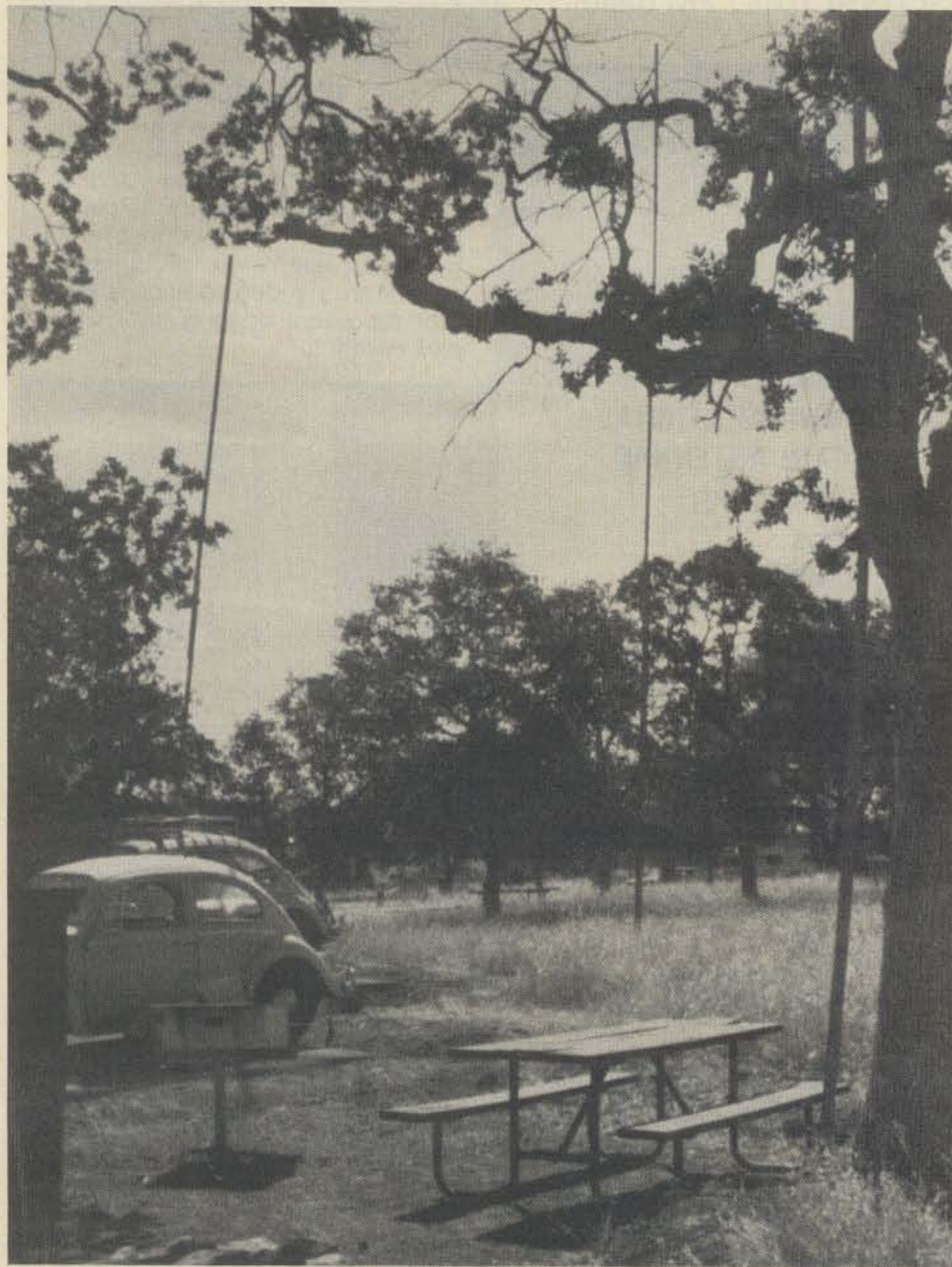
K6TG/6 near Don Pedro Dam, Tuolumne County, Calif. 1976 Field Day. Center 40 ft. pole holding up the apex of the 450 ft. V beam—other two poles for the 67 ft. inverted EII.
