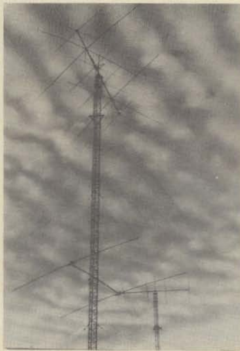
Fig. 9—The K5JA monster Quad with the two element beam below it. In the background is the second 160 foot tower with a wide spaced four element, 20 meter beam on it.
