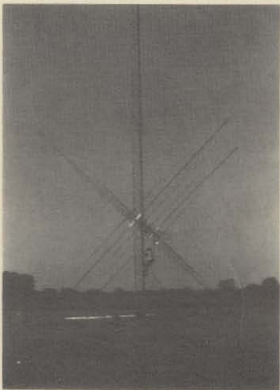
Fig. 5—Final inspection is completed and K5JA returns to ground level. The trick will be to pull the Quad to the tower top without getting entangled with tower guy wires.
