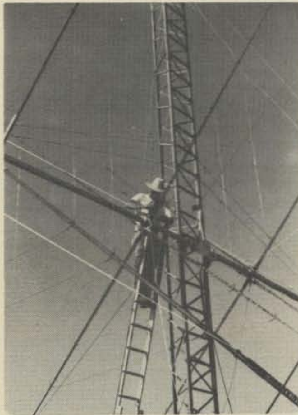
Fig. 2—K5JA putting the finishing touches on the beam. There are six elements on 20, 15 and 10 meters. Boom diameter is three inches and antenna weight is about 200 pounds.
