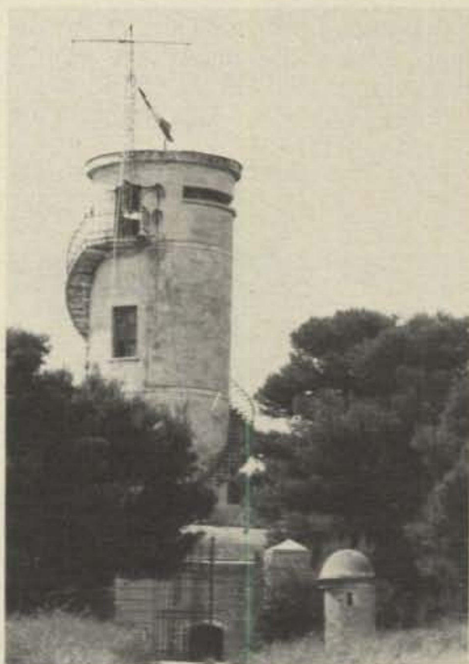
The exterior of IJTEX. On the upper floor of this military tower, the operations took place. The TH3 was fixed on top of a small tower tied to the staircase.
