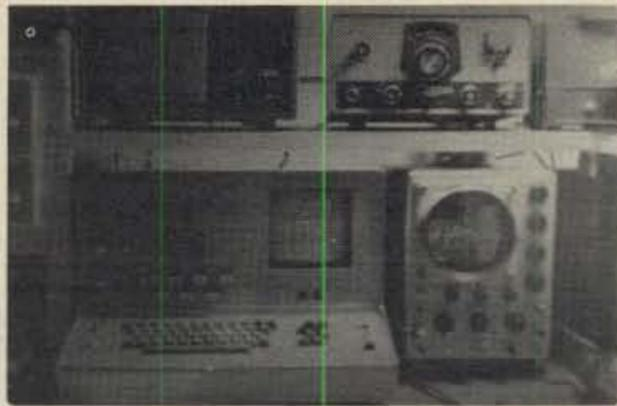
Close-Up view of VK2NM's homebrew combined SSTV monitor and SSTV keyboard. Scope at the right is used for monitoring TV waveforms, etc.
