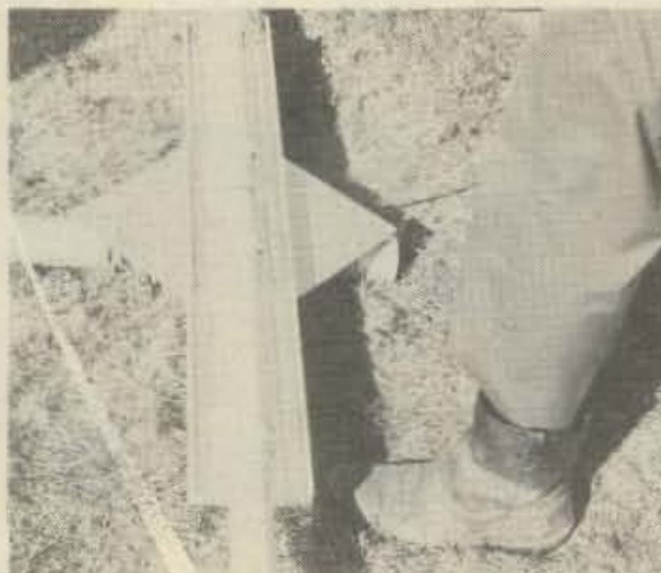
Fig. 7 — The center-point and support for an 80 meter element at K3WX. Note the heavy-duty construction.
