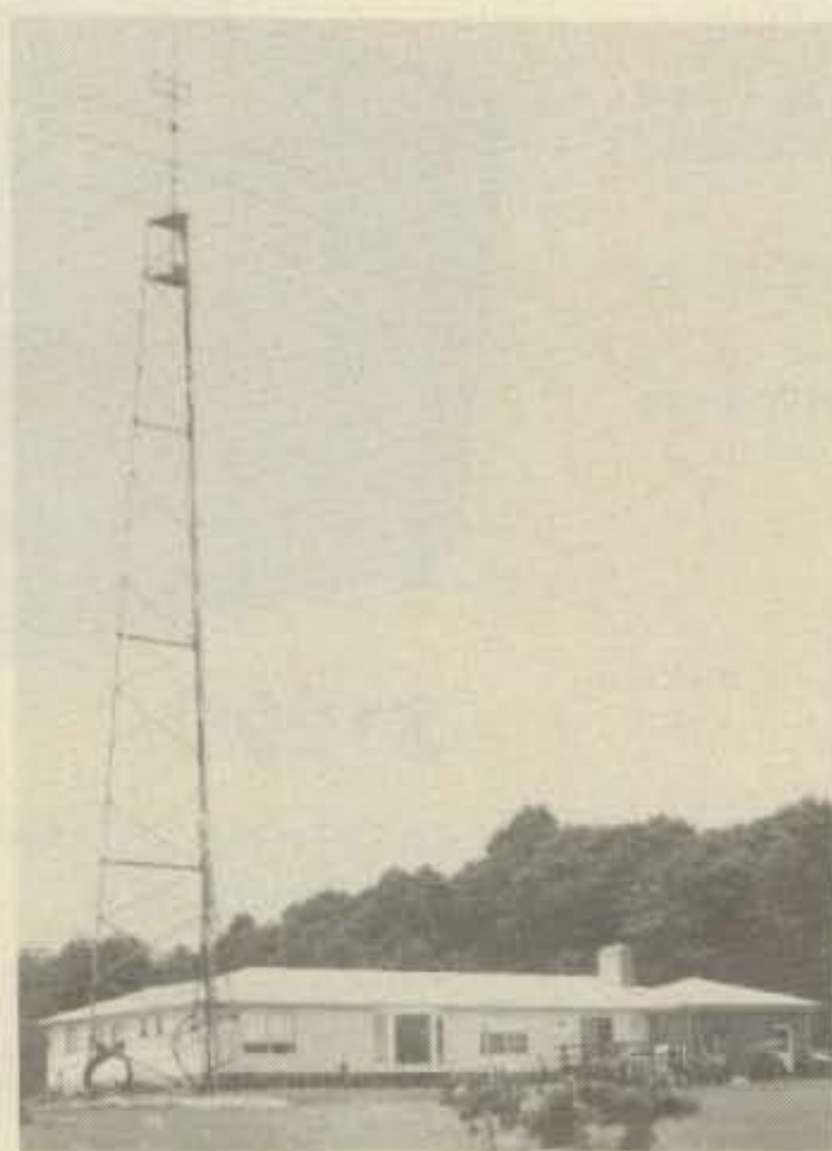
Fig. 2 — The “antenna farm” at K3WX. Tony has a modest 160 foot tower at the side of his house which supports antennas for all bands between 80 meters and 2 meters. There are stacked 20, 15 and 10 meter beams in this view, plus assorted v.h.f. antennas atop the structure.
