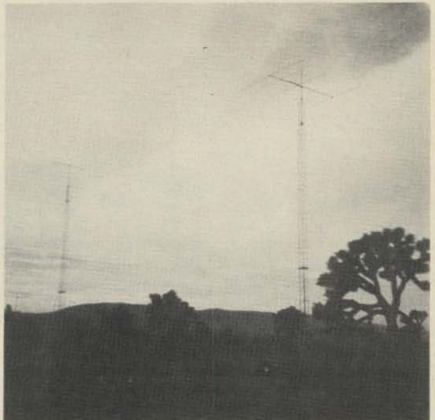
The source of the second highest WIVE single op score, K6SE, a two-element switchable beam on 160. They are "top-loaded" 80 foot towers sitting on 5 miles of radials. Four beverage antennas were used.
