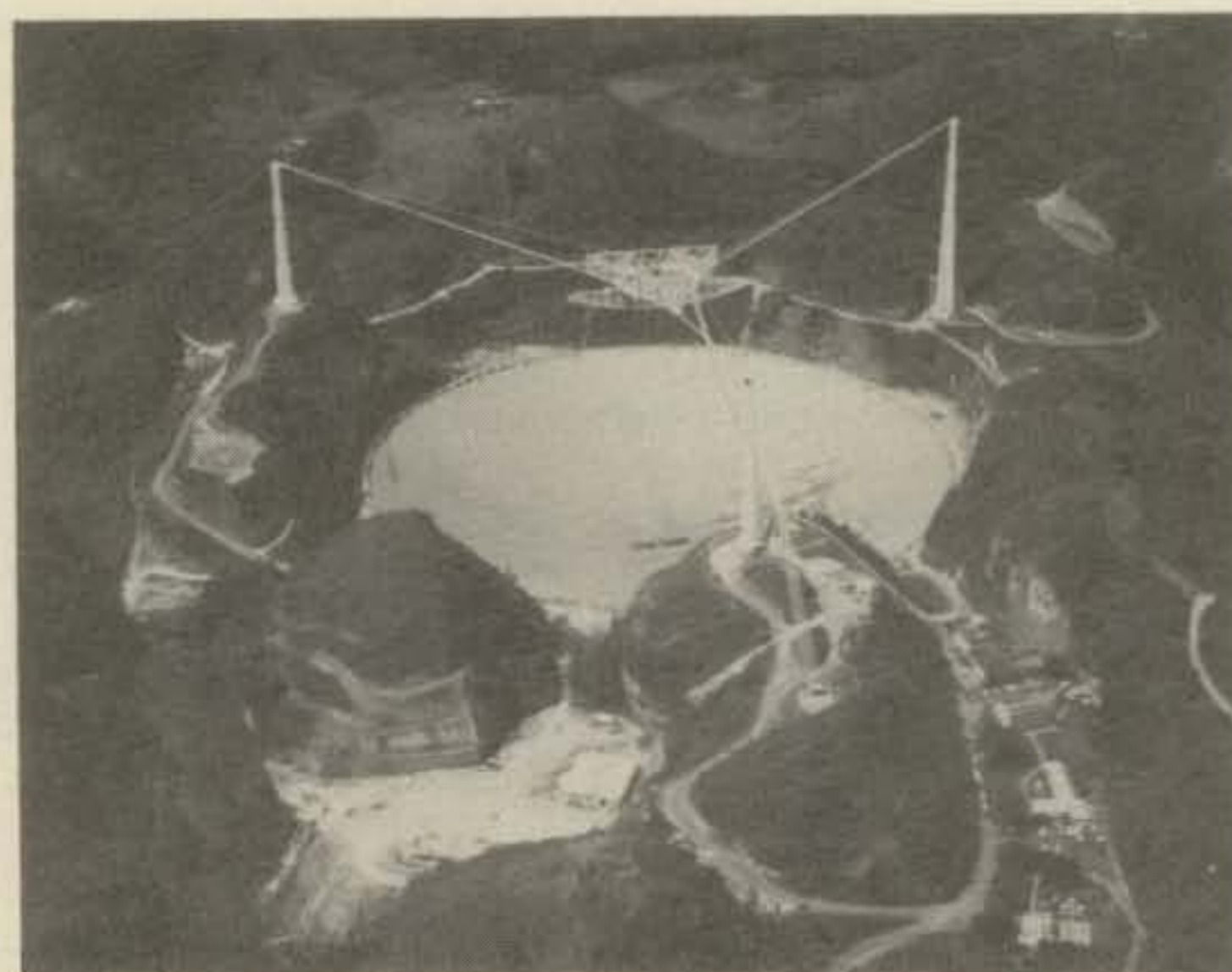
An overall view of the Arecibo antenna. The dish is 1000 feet in diameter. The Arecibo Observatory in Arecibo, Puerto Rico, is part of the National Astronomy and Ionosphere Center, a national research center operated by Cornell University under contract with the National Science Foundation.
