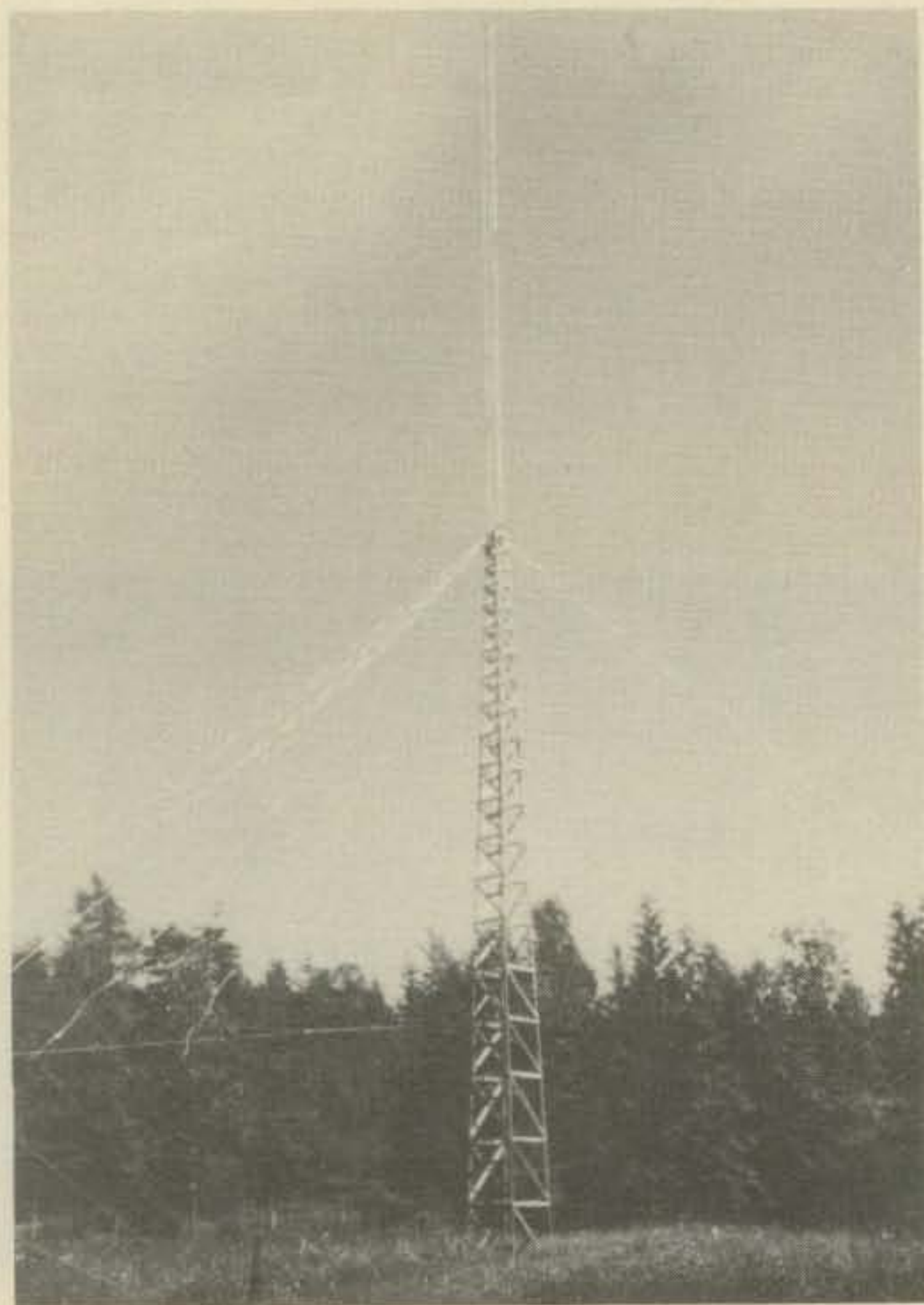
This 80 meter vertical with the top at 118 feet is one of the fabulous 13 antennas at VC7WJ.
