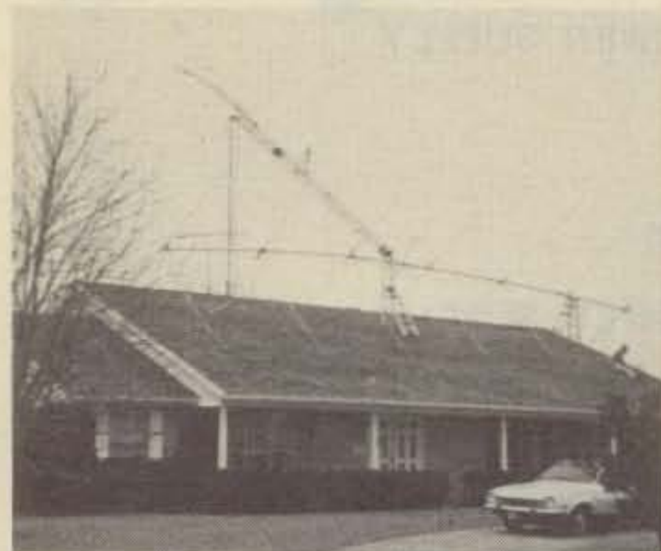
Fig. 1 - The "Monster Quad" of W5MOK folded over for maintenance. This array has seven elements for 10, 15 and 20 meters on a 62 foot boom. A stepladder on the roof of the house allows easy maintenance.
