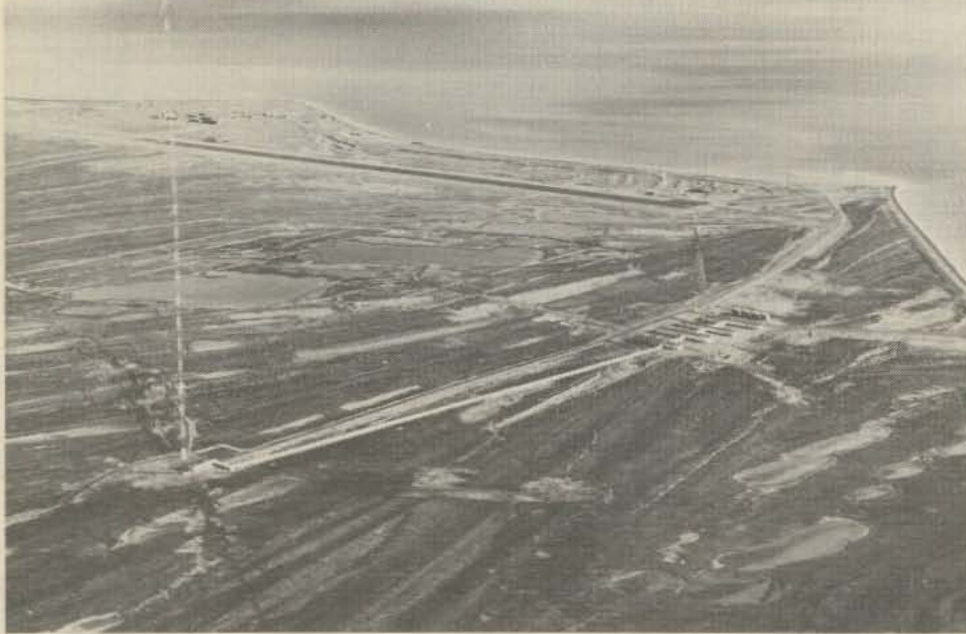
Poised high above the terrain at Port Clarence AK, this 1350-foot top-loaded vertical is part of the North Pacific Loran-C chain operated by the U.S. Coast Guard. The 100 kHz transmitter puts out nearly a megawatt of power.
