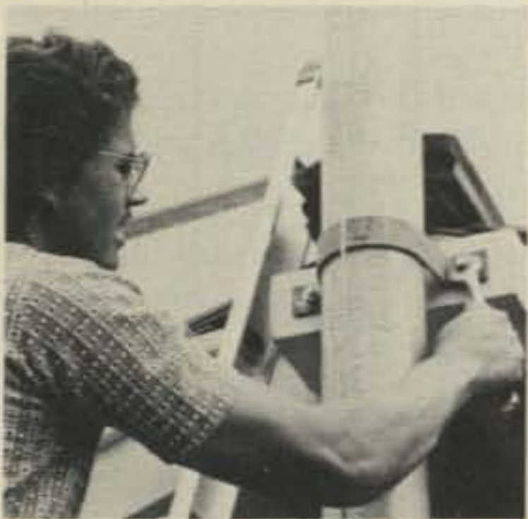
Mounting the House Bracket
