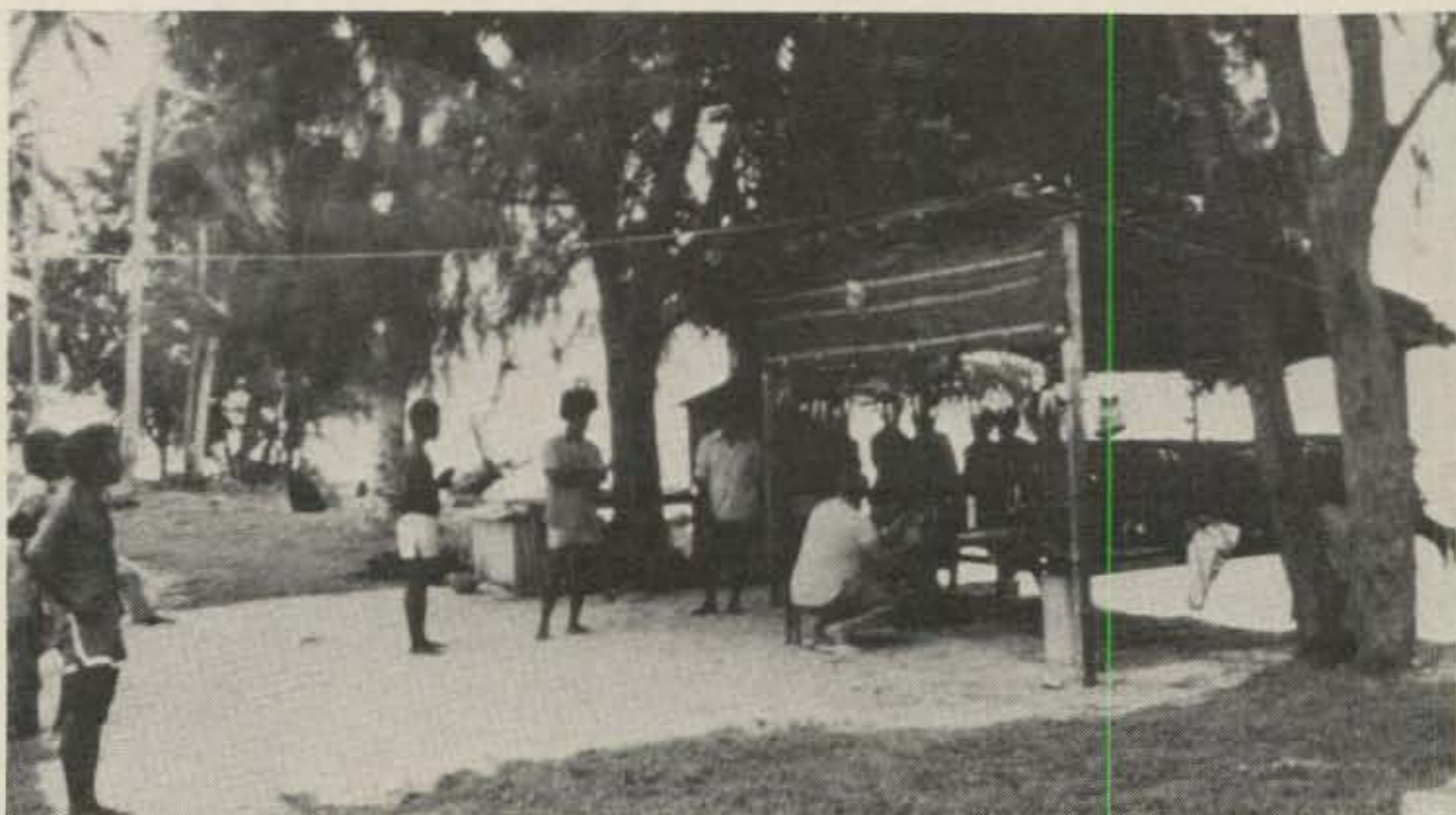
The radio shack on Kat Island.
