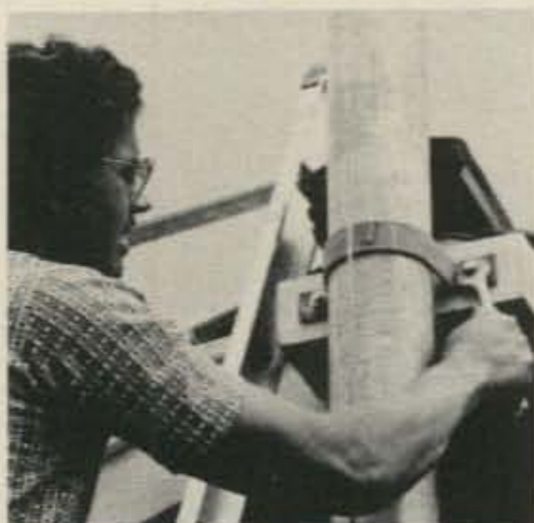
Mounting the House Bracket
