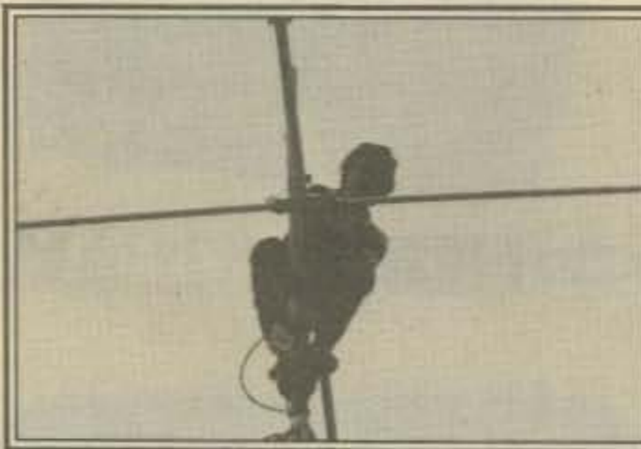
Torros, A7XM, has given many DXers a new one from his QTH in Doha, Qatar. In this photo he is installing a new TH6DXX at 45 meters. QSL A7AM via DJ9ZB. (Photo courtesy DJ9ZB)
