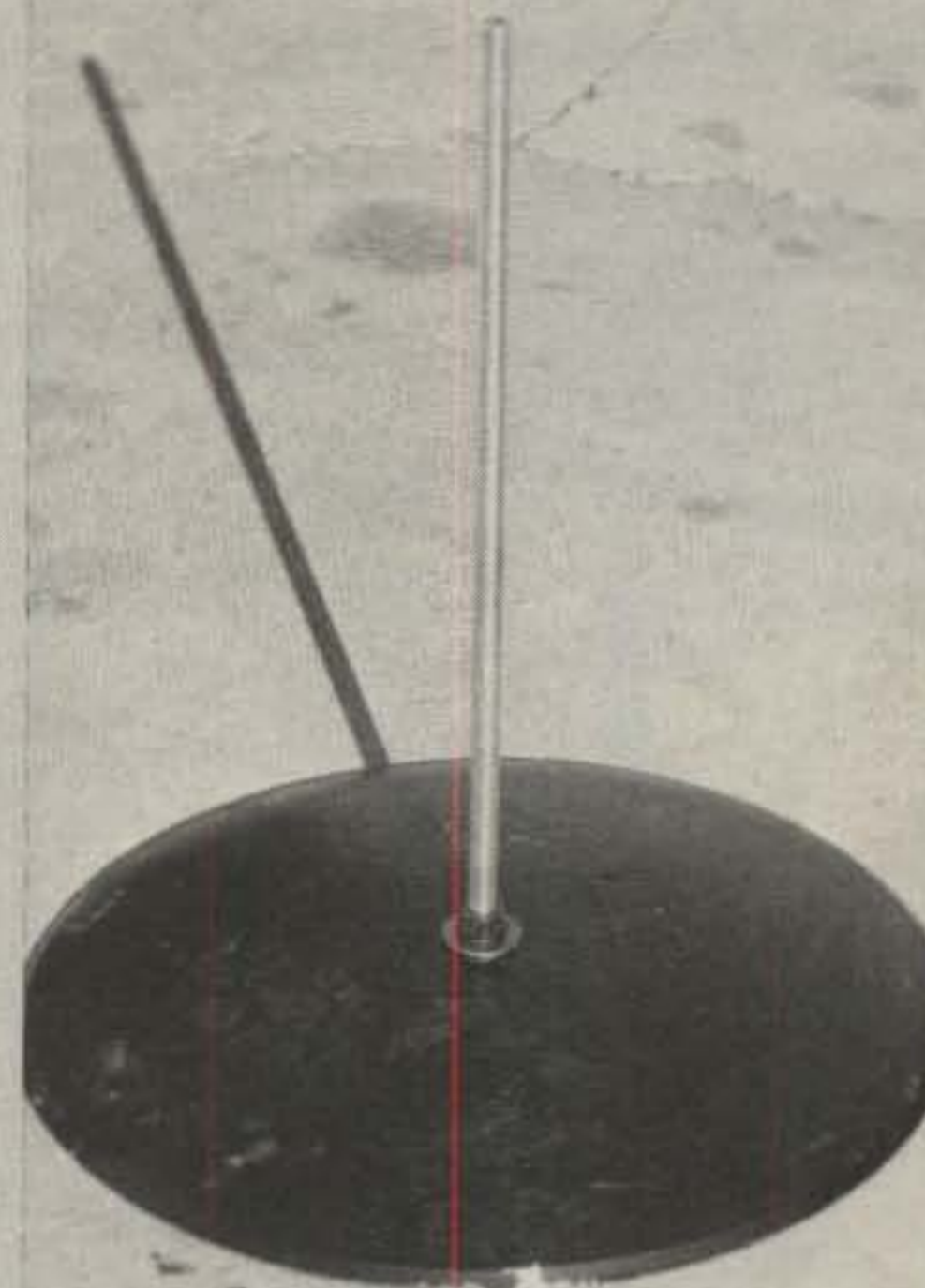
Fig. 2- Mounting the vertical antenna at the center of the mobile home roof.
