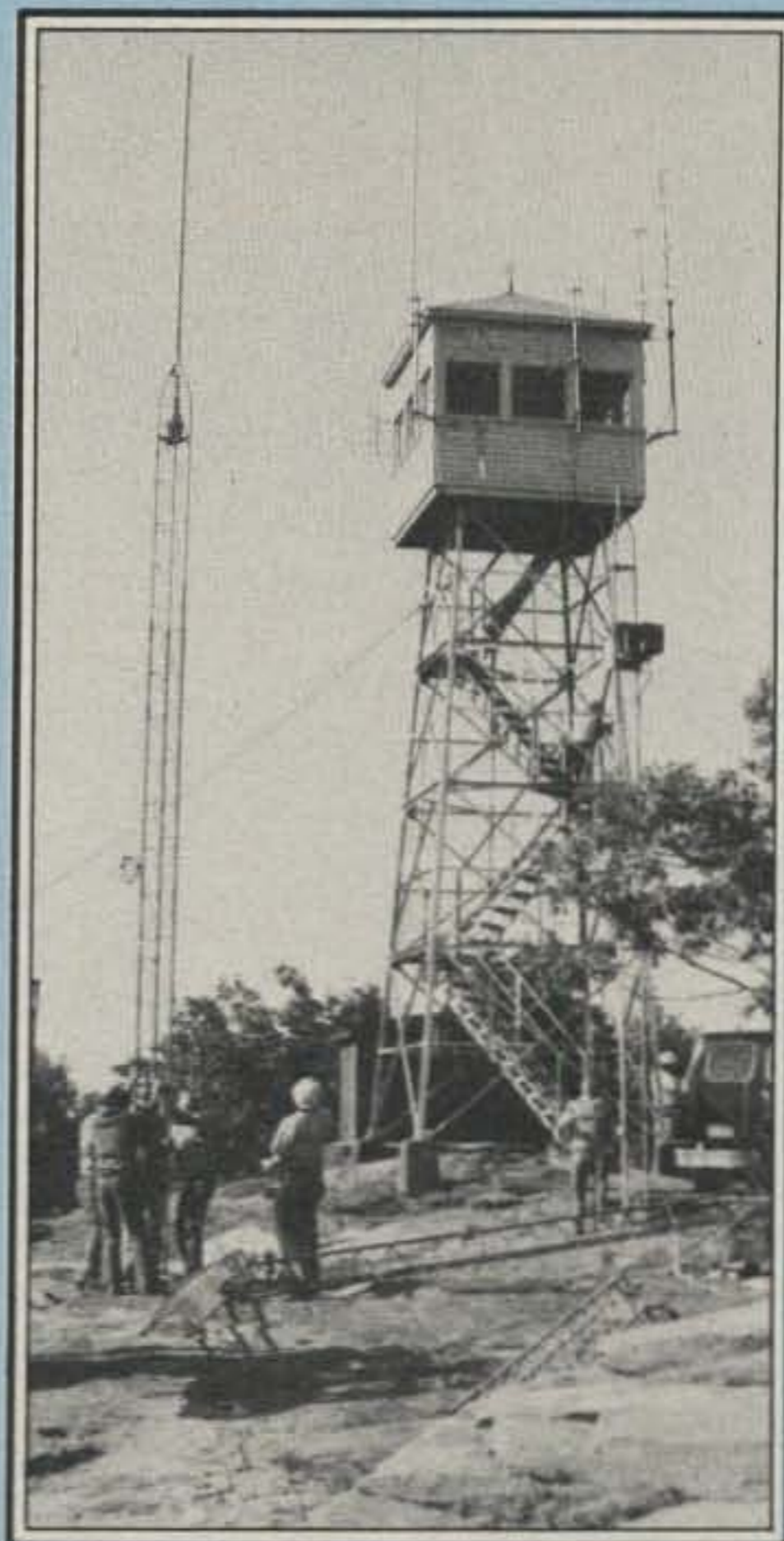
Erecting the tower next to the ranger station.
