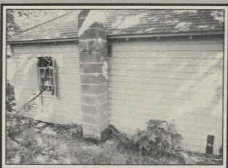
The power installation.
