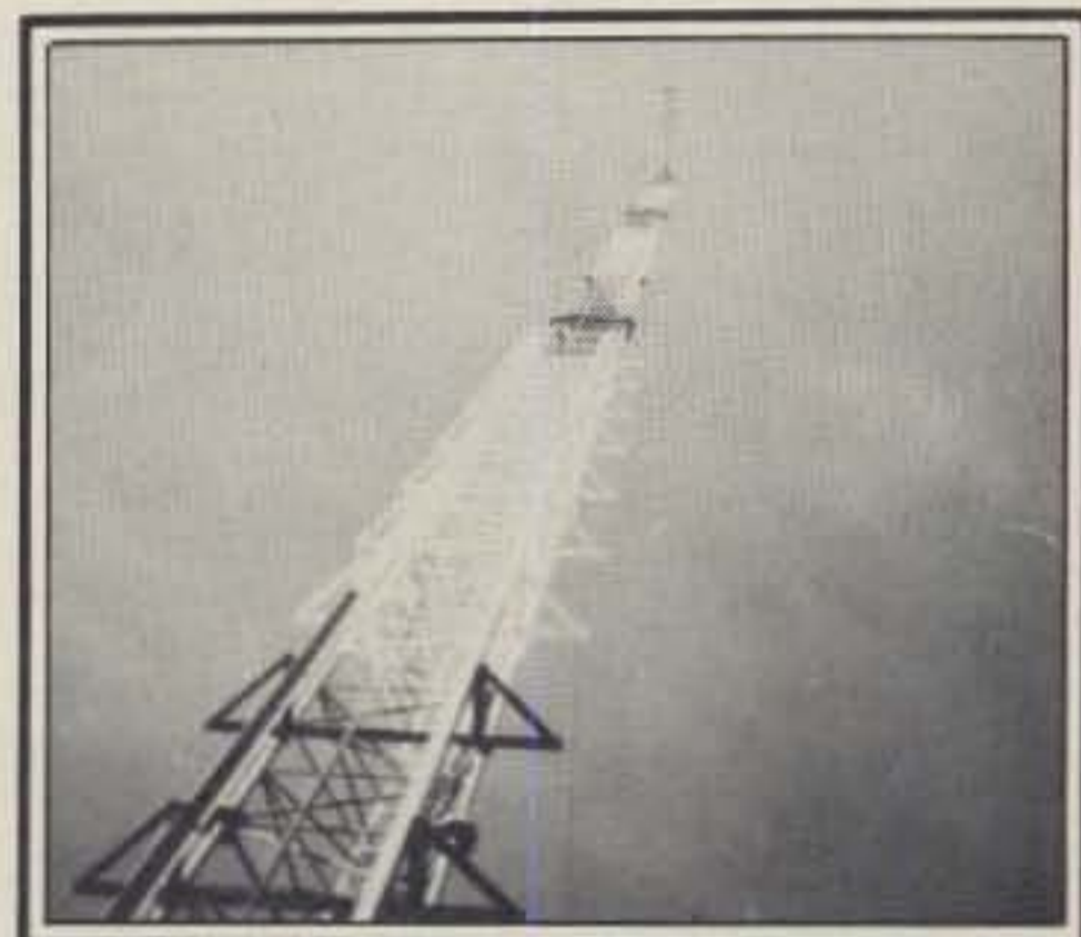
Shown here is one of the 400-foot WWVB and WWVL antenna towers; the antennas are identical, and are top-loaded. Both stations are sister installations to the familiar h.f. time-ticker, WWV, though the 20 kHz WWVL transmitter has not been on the air regularly since 1972. The 60 kHz WWVB station is extensively used, however, to provide good coverage of the entire continental U.S.A. with precise time and frequency data much in the same way that WWV provides consumer-type calibration information on popular h.f. frequencies (5, 10, 15 MHz, etc.). The bandwidth of the WWVB antenna is about 600 Hz, while the bandwidth of the WWVL antenna is but 20 Hz! Not surprisingly, efficiencies are low; 35% for the 60 kHz WWVB antenna and 5% for the 20 kHz WWVL antenna. Shades of 75-meter mobile operation!
