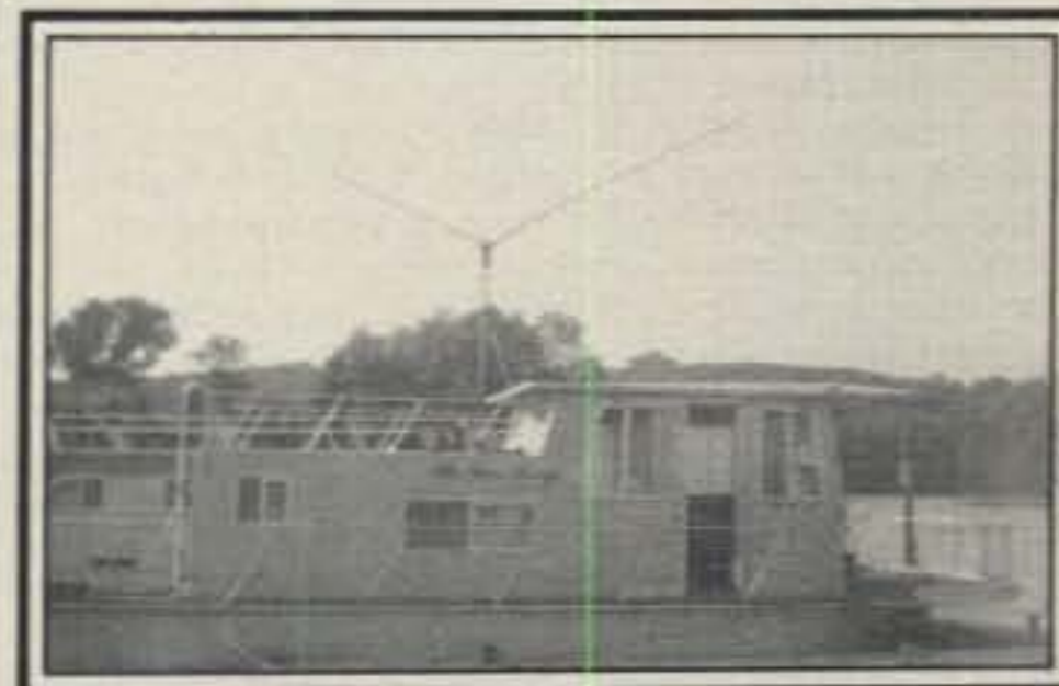
The K4OU site. The moored "The Love Barge" sporting the 10-15-20 meter dipole fabricated from a pair of 12-foot collapsible fishing poles. Despite the low height of about 12 feet above water level, the antenna performed excellently at 176 QSOs.
