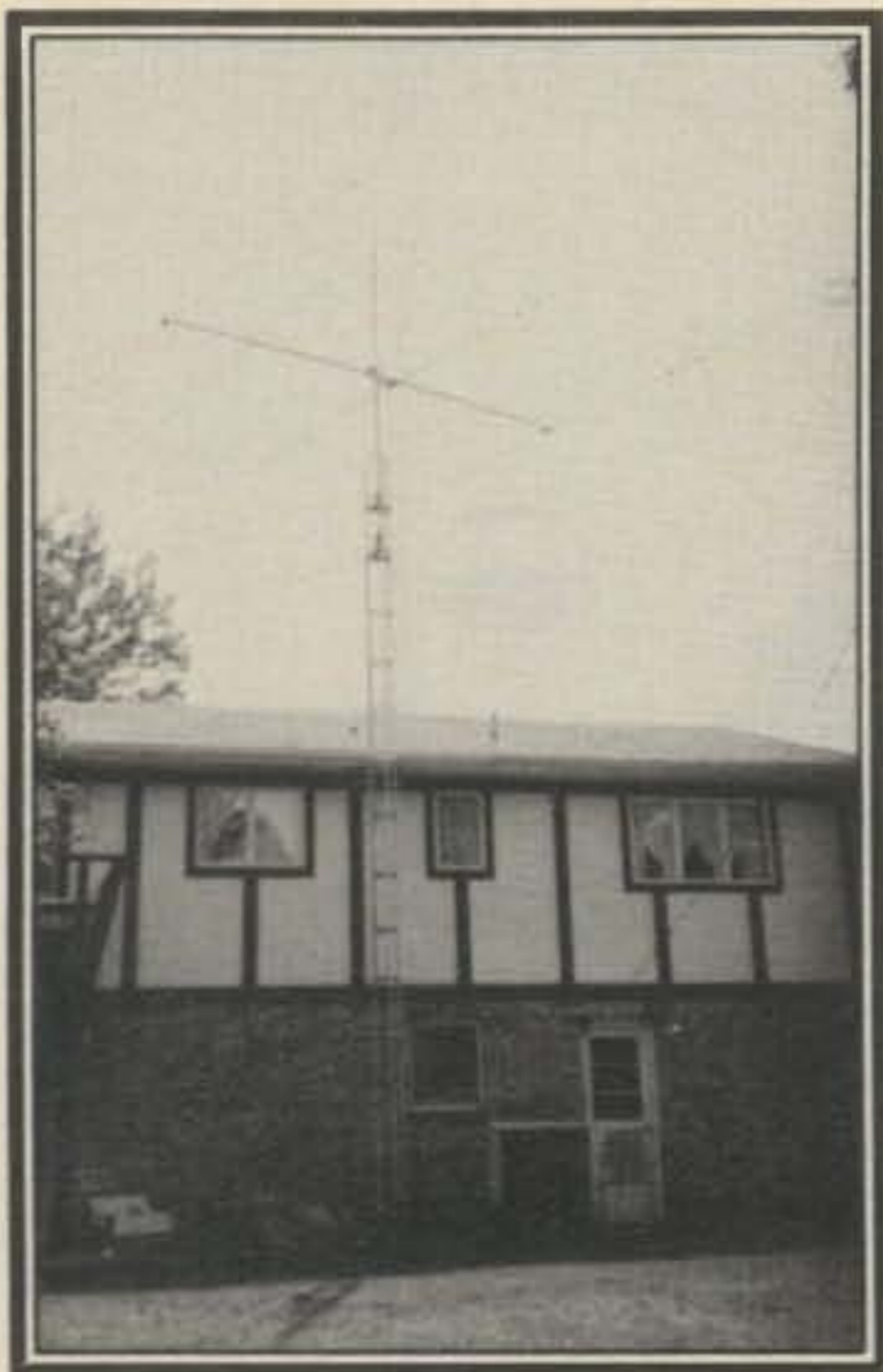
The tower with the beam and Ringo Ranger mount to the back of the author's house.
