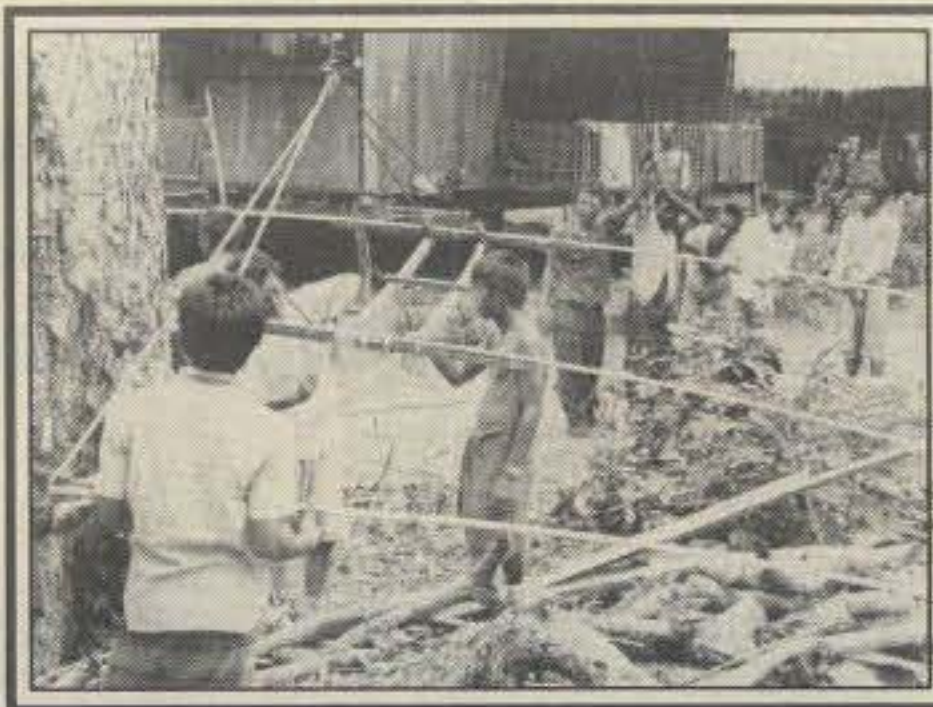
JA8BMK and other members of the crew working on the 14 MHz 3-element yagi.
