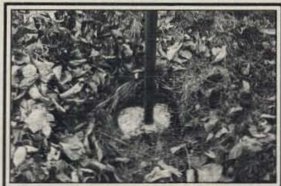
Here the leaves are brushed aside to show the base plate for the "tap-in" tapered in-ground mount.
