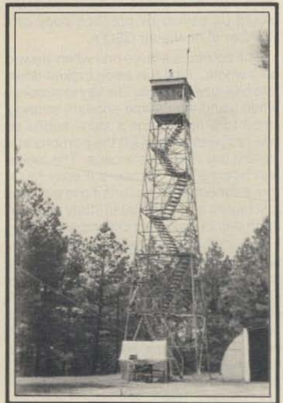
The fire observation tower, with a 16-element 144 MHz yagi on top at Woodall Mountain (the highest point in Mississippi). This antenna helped W9IP/5 work 27 ARRL sections on 2 meters in the September 1980 ARRL VHF contest.
