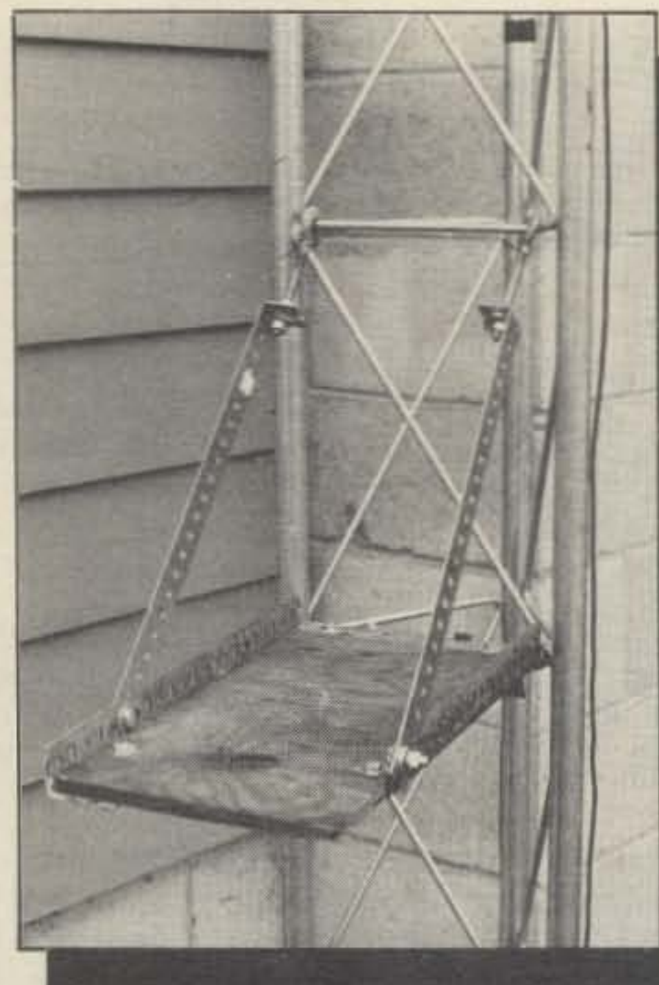
Working platform assembled. Forged hooks were used at the top of the supporting braces, and safety wire was used to secure hooks to the tower crossmember.
