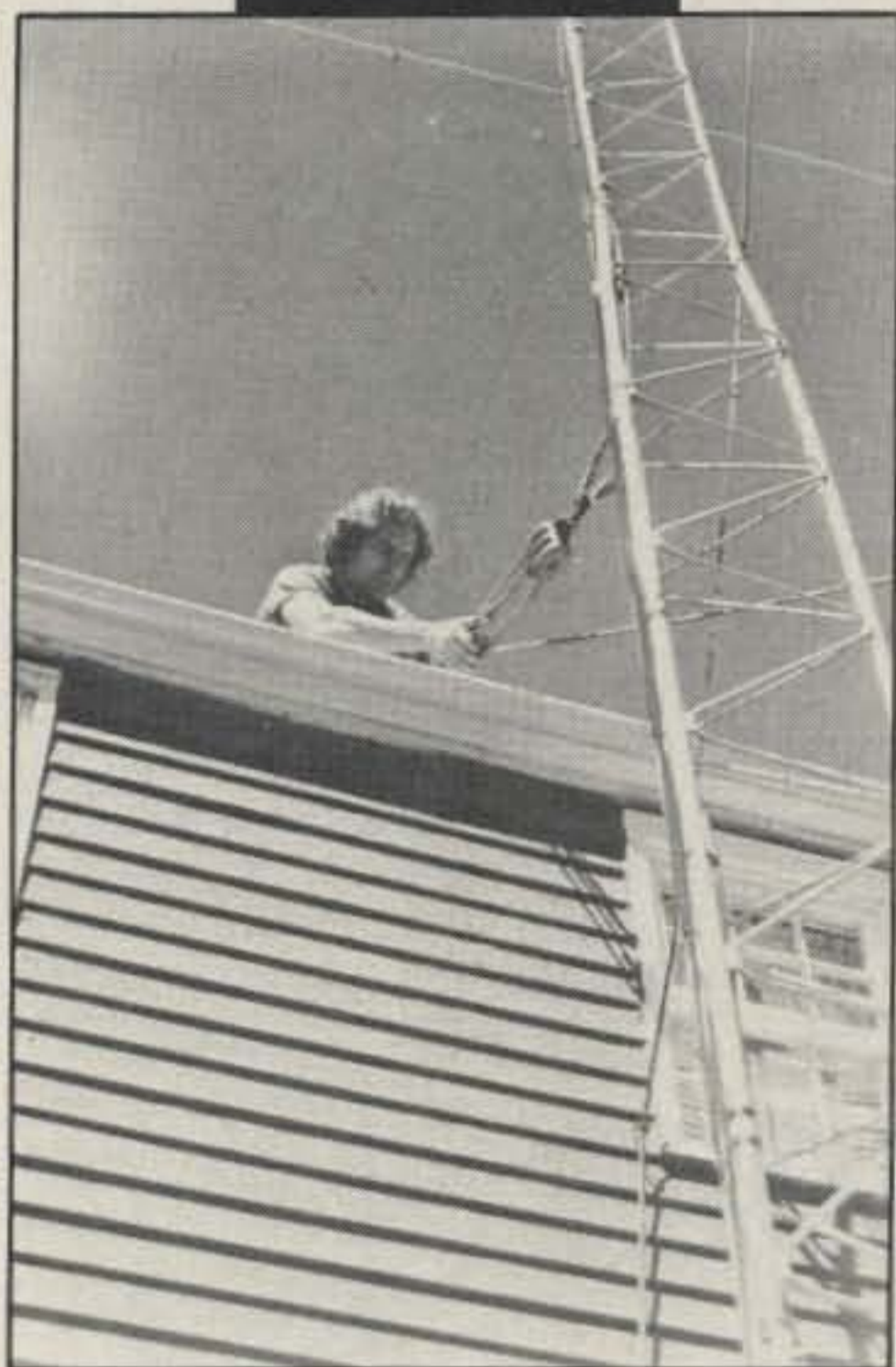
WB1GIF checks the block and tackle prior to lowering the tower to replace the beam and rotor.
