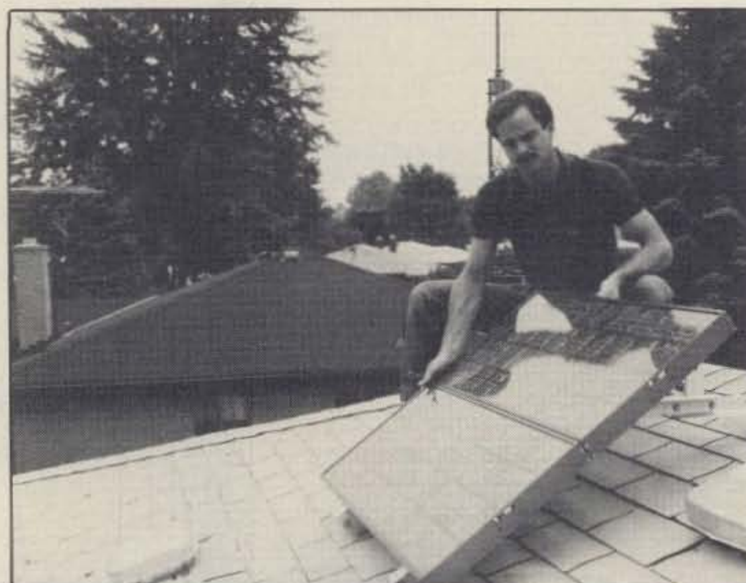
Here is WD8AHO installing the panels on the roof.
