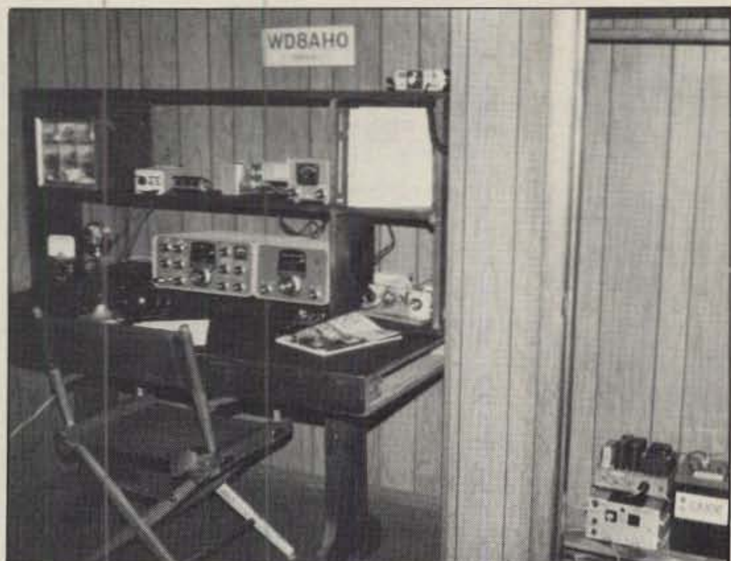
This will give you an idea of what a solar-power amateur radio station looks like (except for the panels on the roof).
