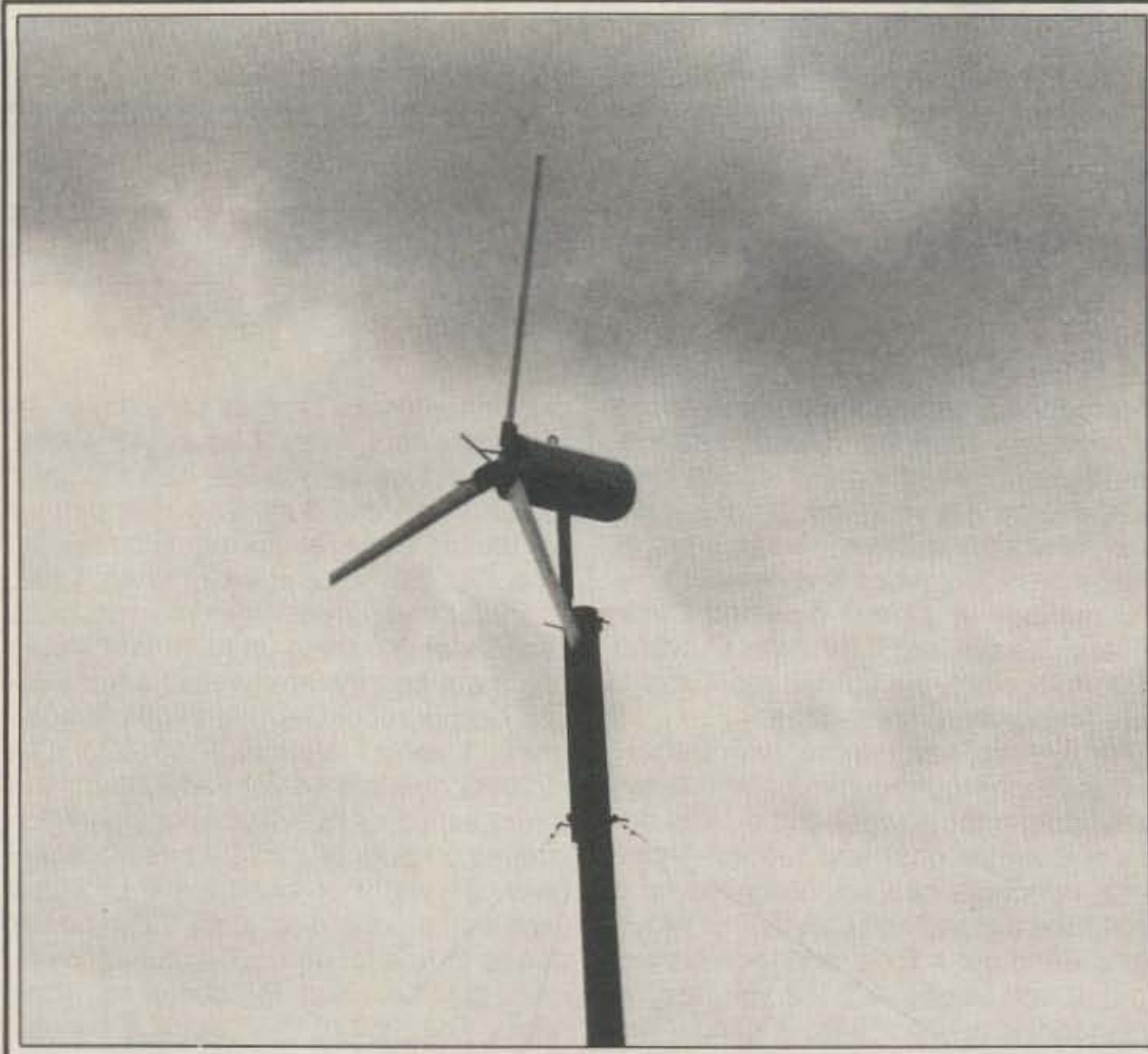
Neat, clean, and effective, this Windpower Corp. wind generator provides up to 1500 watts of usable energy. Installation is less trouble than erecting a triband beam.
