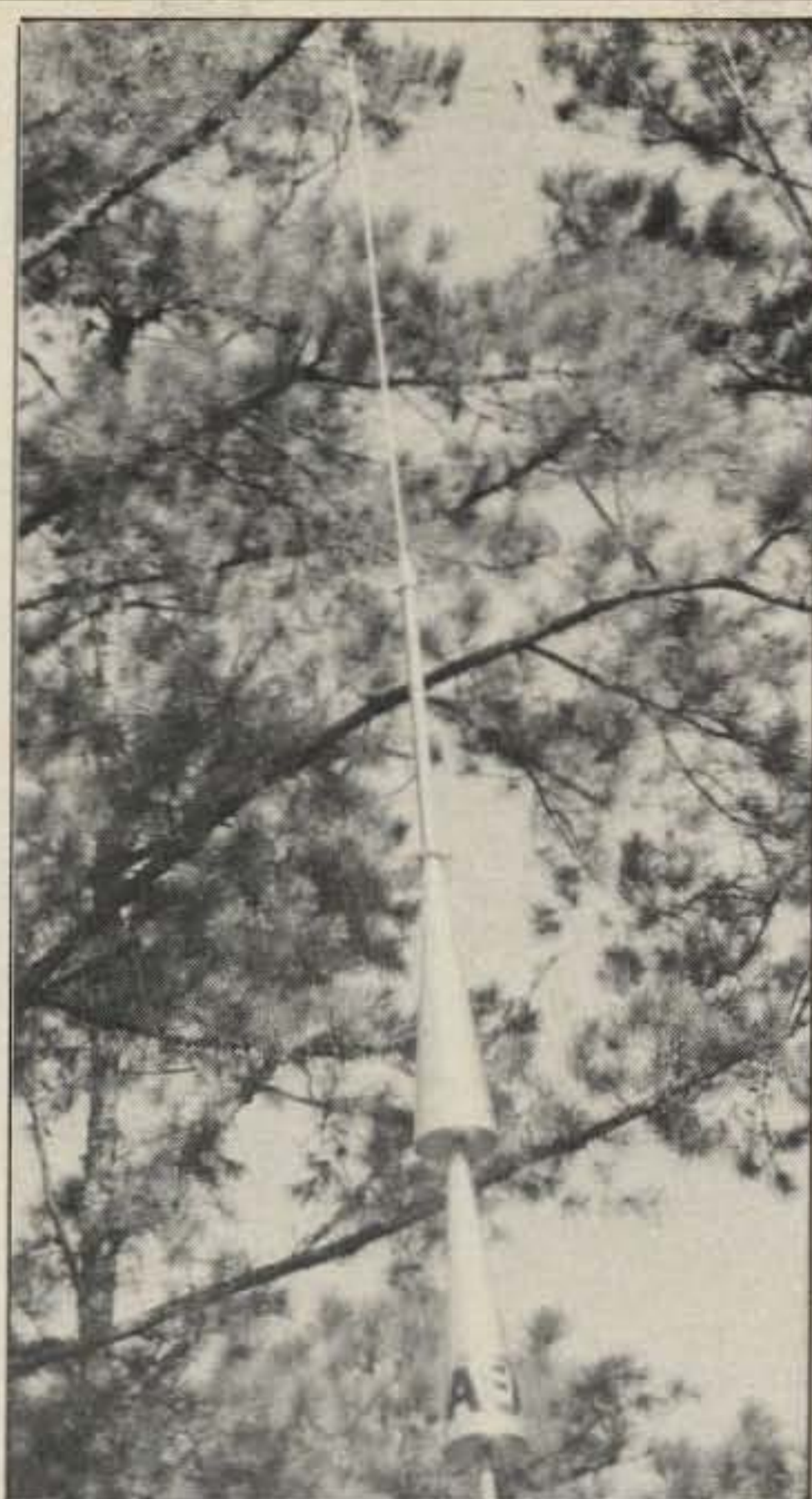
A close competitor to the Butternut Trombone is AEA's IsoPole, shown here in the author's installation. Line decoupling is a major design feature of the AEA vertical. (W8FX photo)
