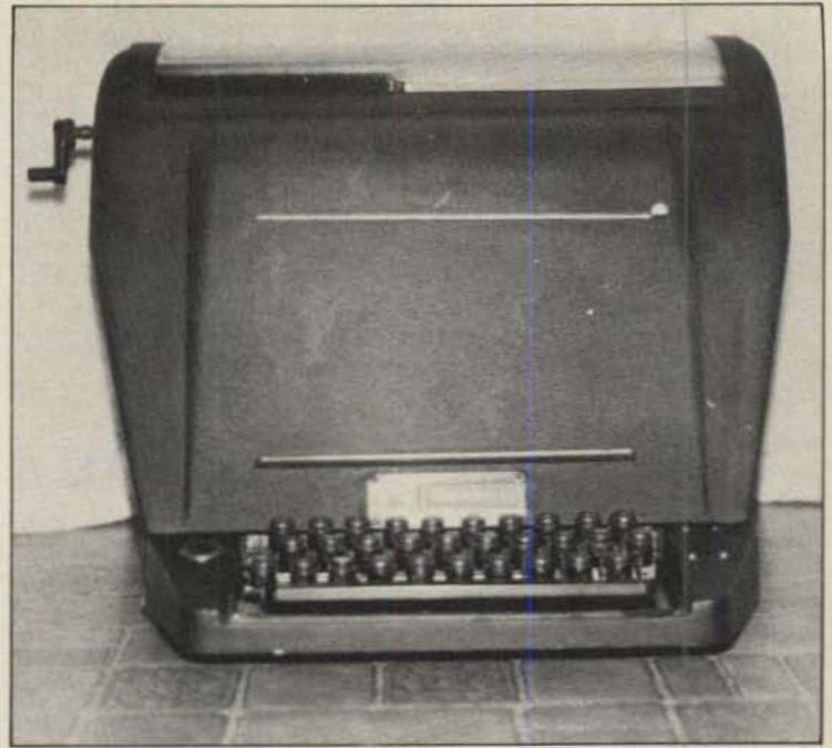
The classic model 26 teleprinter was a quiet and compact unit designed primarily for light-duty operation. The unit still can be enjoyed with today's RTTY setups. (Teleprinter courtesy of Joe Graffo, KA4BDI)
