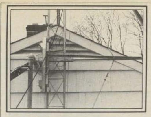
Side view, hinge plate and A-frame structural arm.
