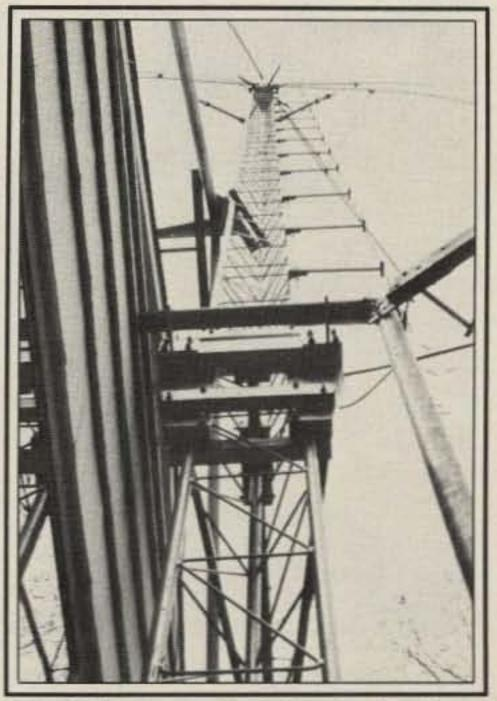
WB3GXV tower showing back side of hinge plate pad.
