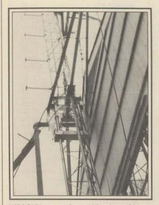
WB3GXV tower, front side view of hinge plate pad with A-frame structural arm.
