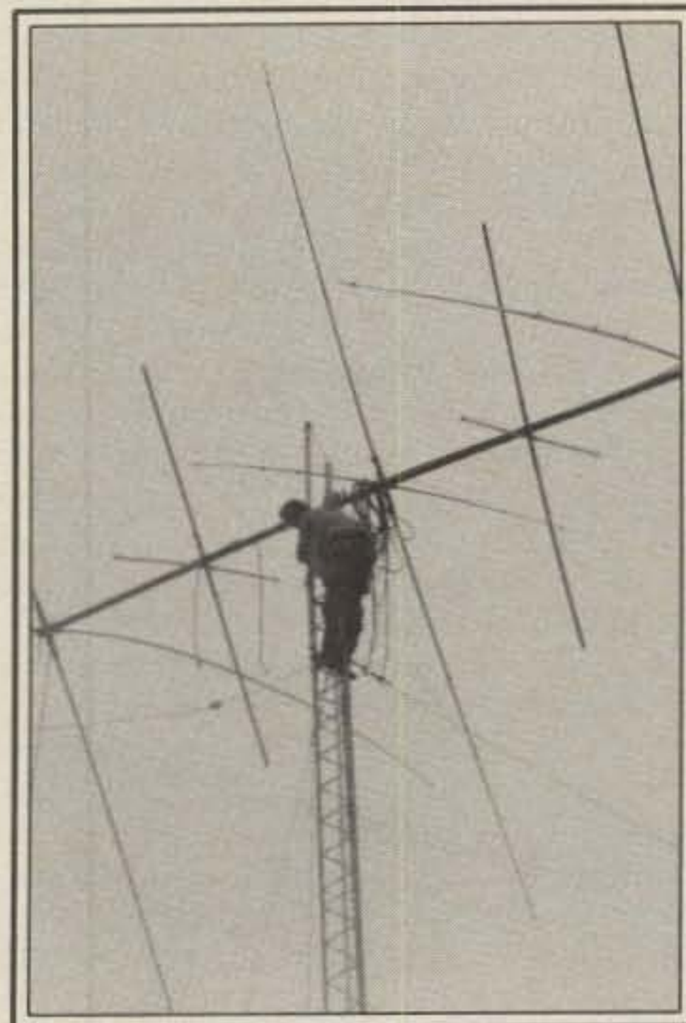
At the top at last! The transition from rail to mast is taking place.
